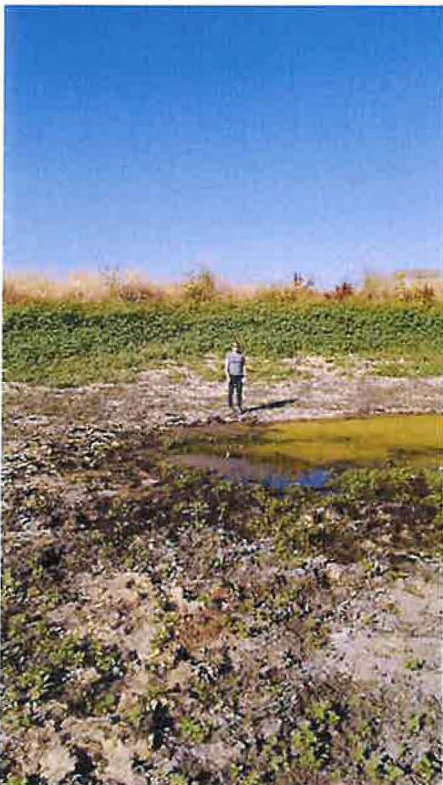
Downstream side of the pond showing the maximum depth of 9 feet.
