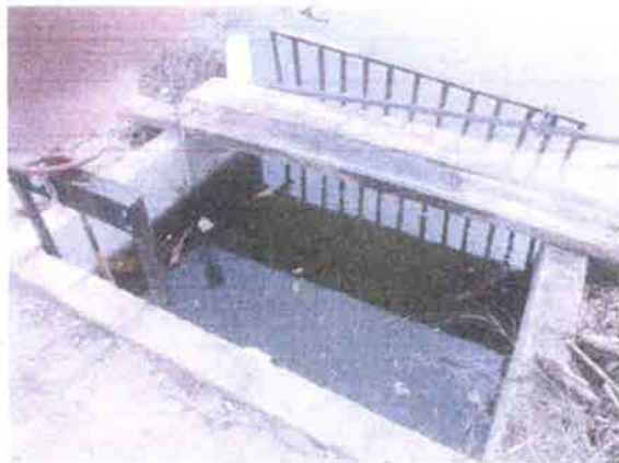
Looking upstream through box.
