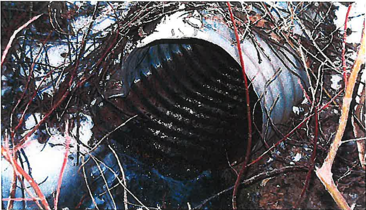
3. Allen Ditch culvert under W. Mtn. Road (Downstream side)
