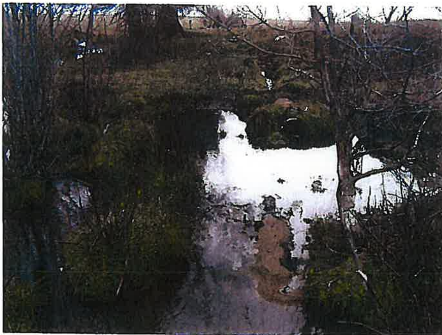
Chess/JR Allen Complaint 11/18/2010 Photo #2: POD for southside acres of right 65-3111X. Water diverted from Rock Ck "Richard's Ck" (foreground and far left of picture) via rusted culvert pipe and ditch (middle ground right of picture).
