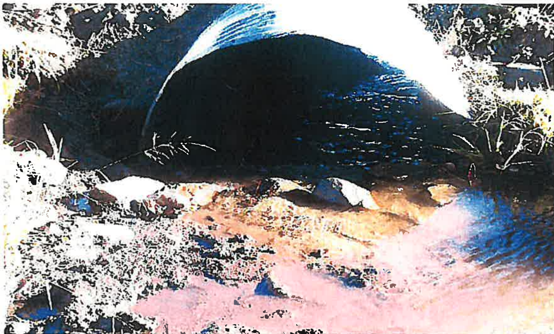
5. Allen ditch Culvert Weir Board northwest of pasture gate
