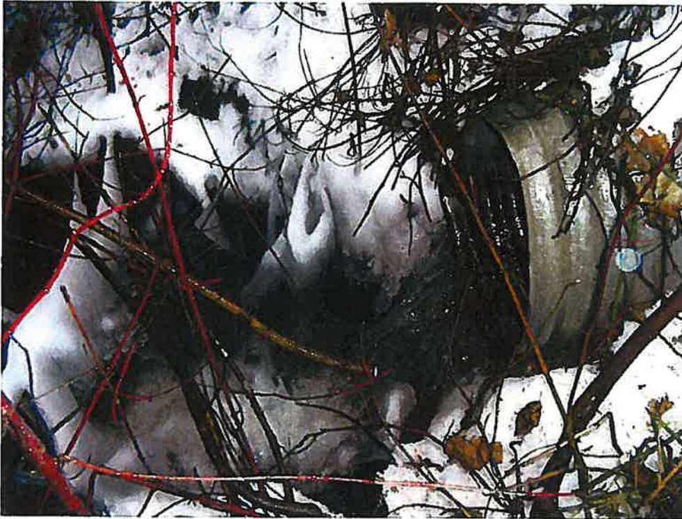
JR Allen Site Visit 11/17/2011 Photo #1: Allen Ditch culvert underneath West Mountain Rd, downstream side.
