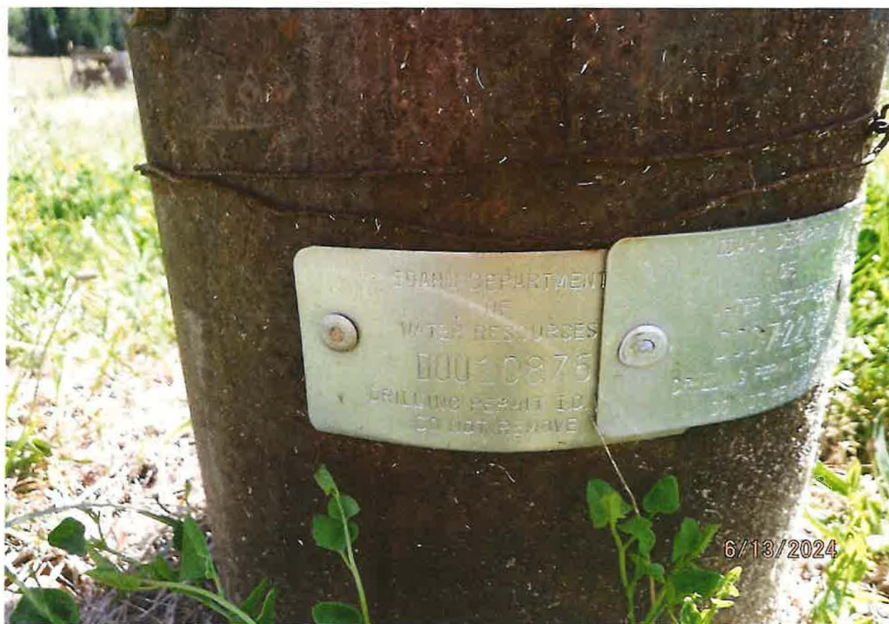
TWO WELL TAGS WELDED TO CASING OF GROUNDWATER WELL
