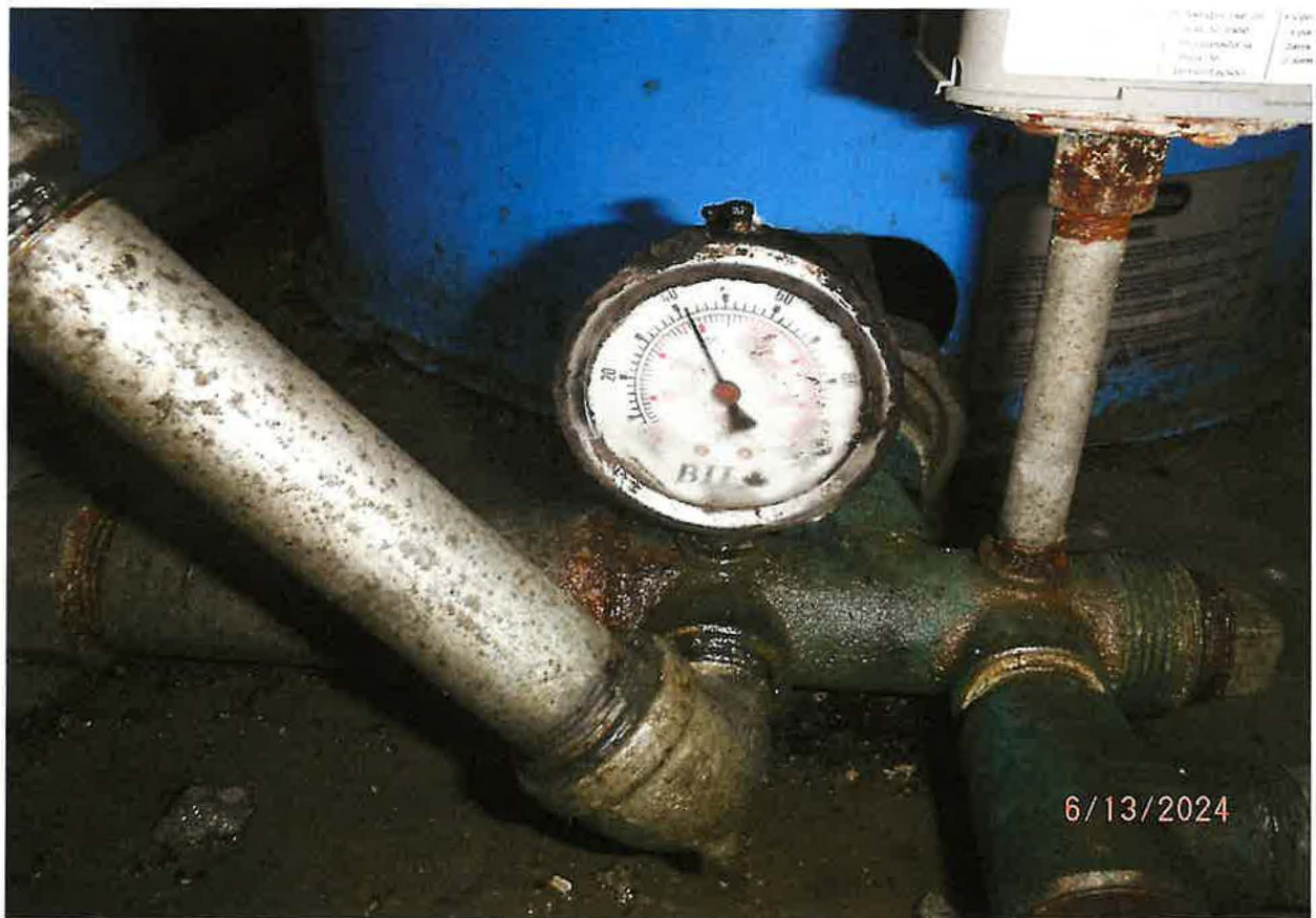
WATER SYSTEM HOLDS STATICALLY AT 40 PSI
