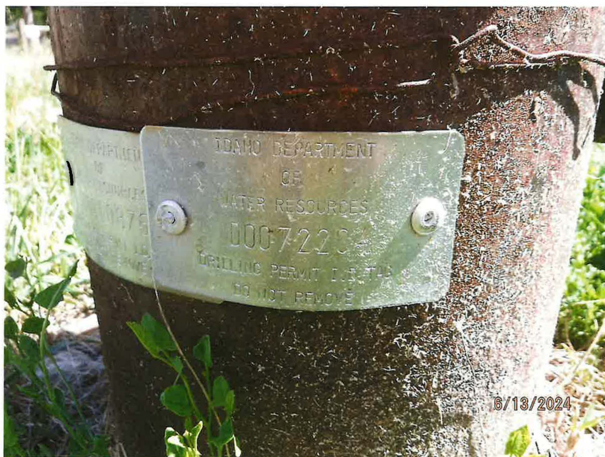
TWO WELL TAGS WELDED TO CASING OF GROUNDWATER WELL
