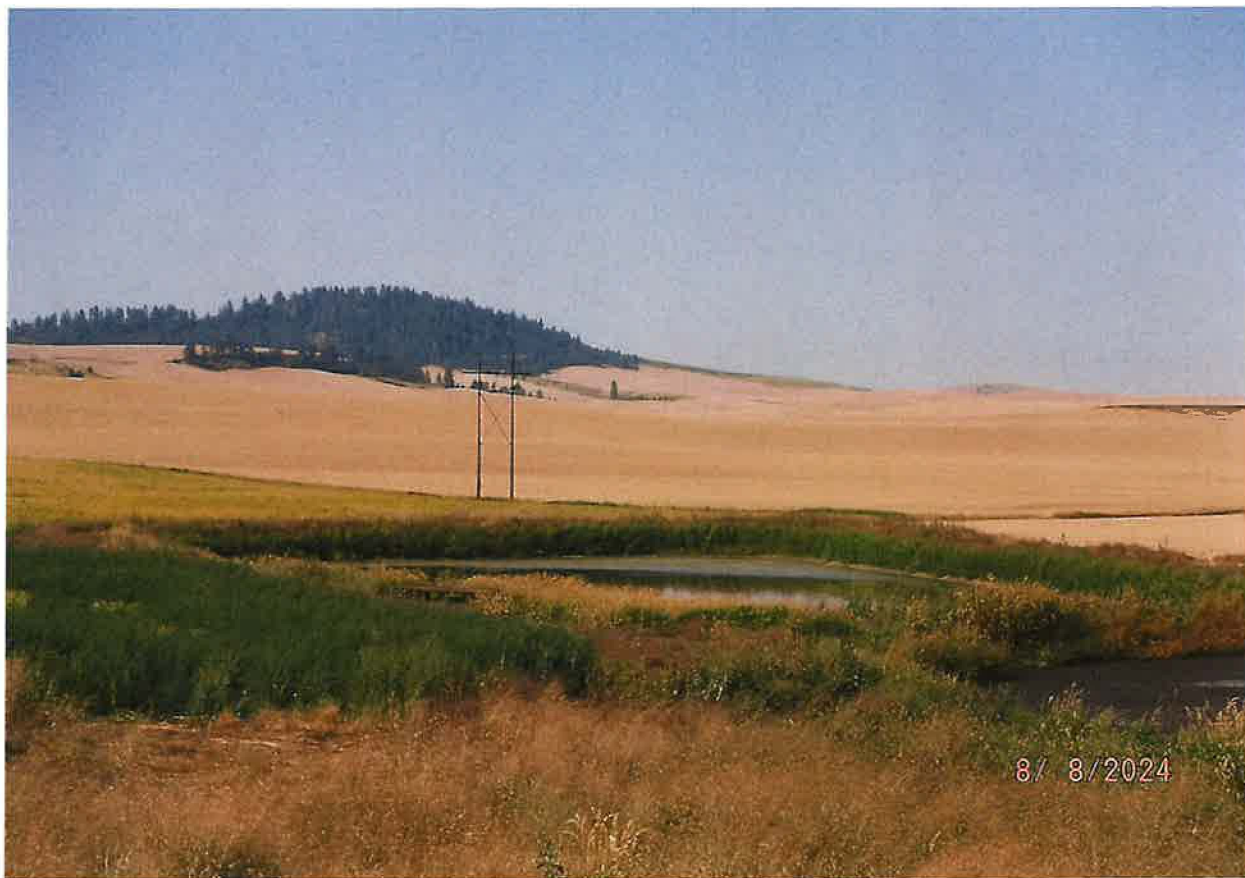
LOWER WASTEWATER STORAGE POND – RECYCLED PUMPING TO SOLIDS POND USED DURING FERTILIZER SPRAYING PRACTICES. REPURPOSING OF WASTE WATER
