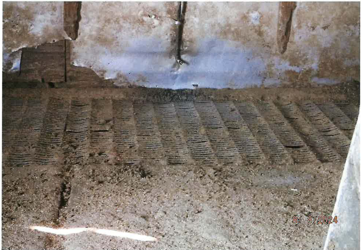
3-FT X 3-FT DRAIN CHANNEL
