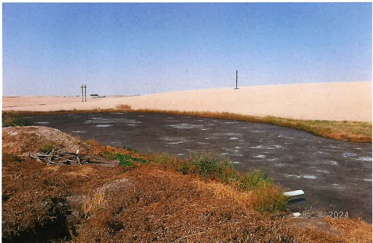
UPPER (SOLIDS) STORAGE POND RECEIVES WASTEWATER FROM STOCKWATER & INDUSTRIAL USES
