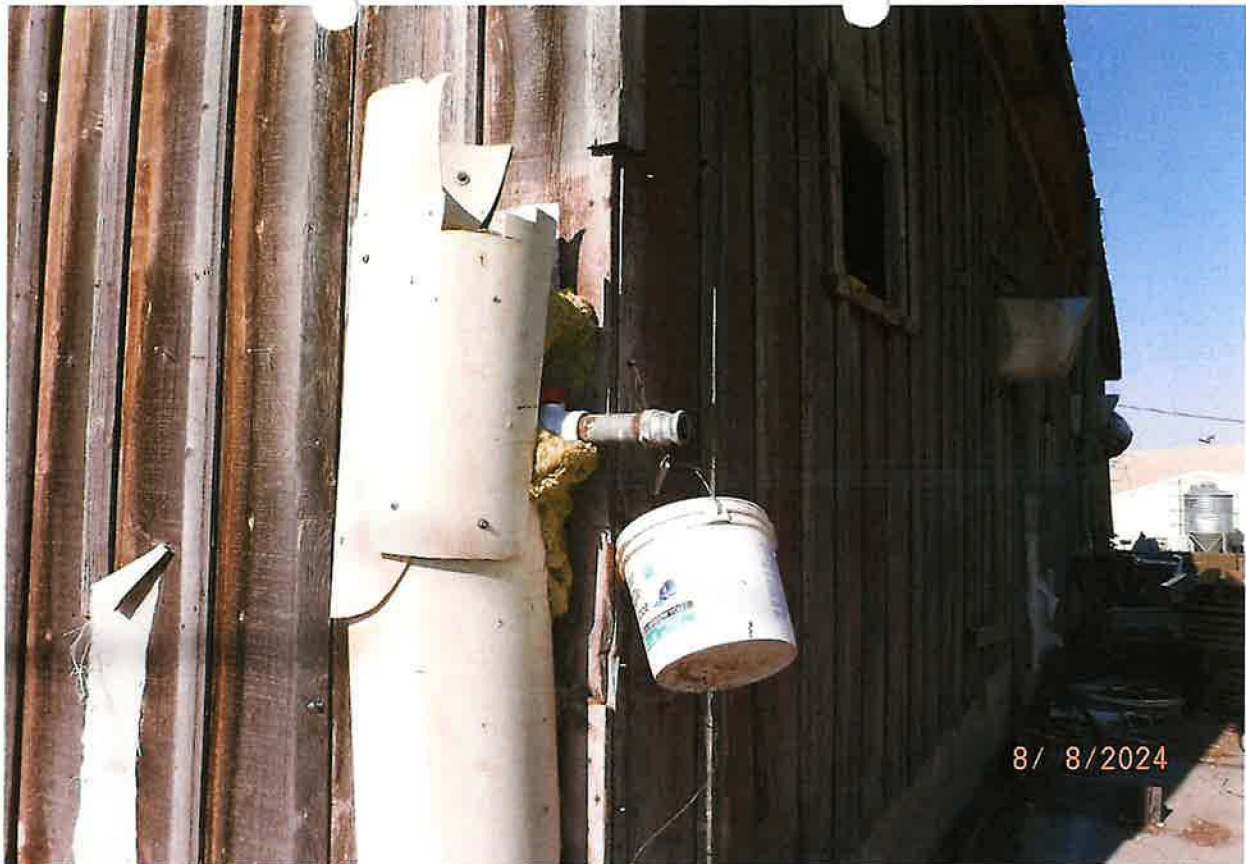
EXAMPLE WATER RISER PIPE ROUTED FROM MAIN MANIFOLD WITH QC CONNECTION TO PRESSURE SPRAY HOSE
