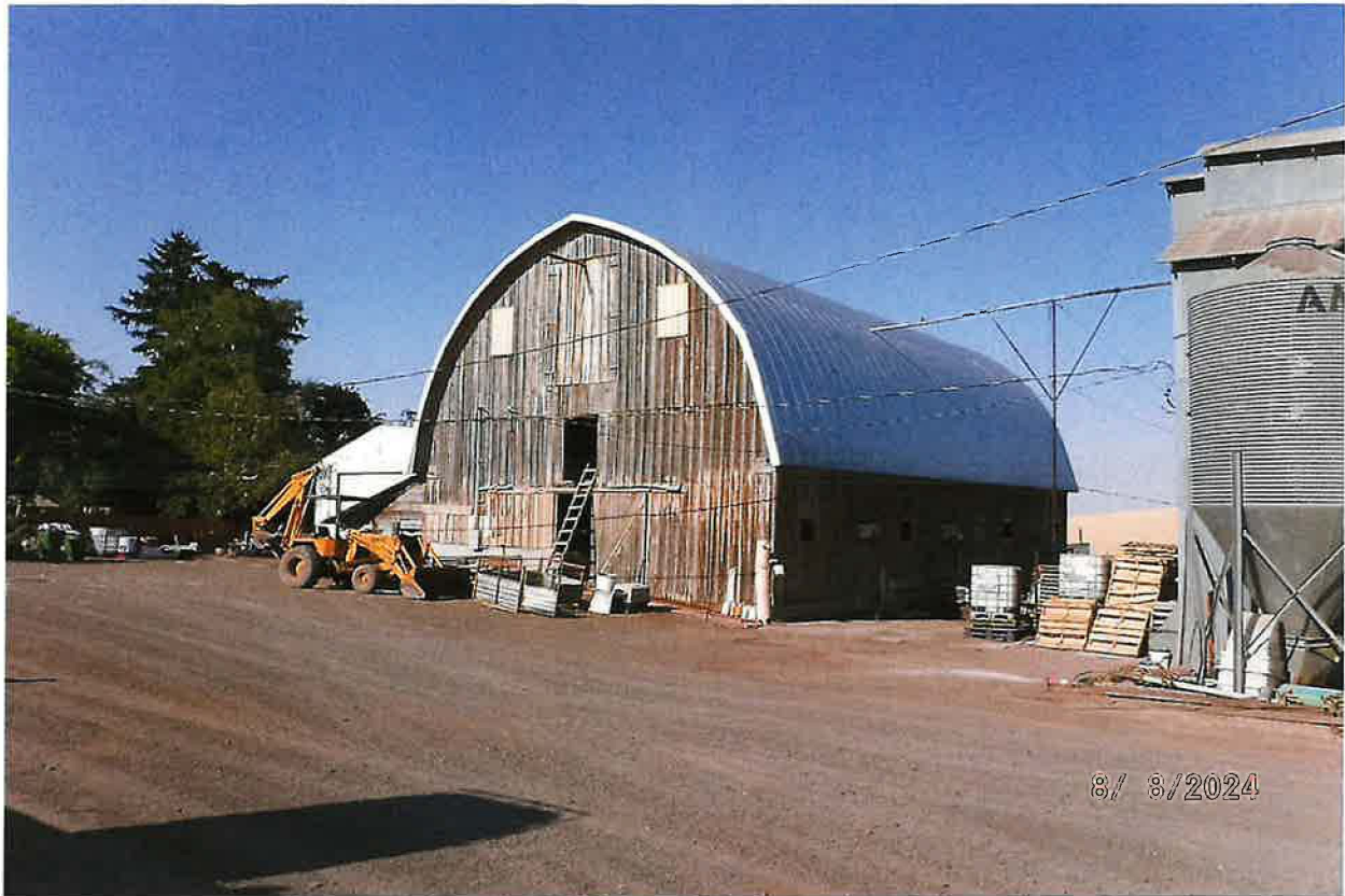
STOCKWATER & INDUSTRIAL POU (GROWING BARN)
