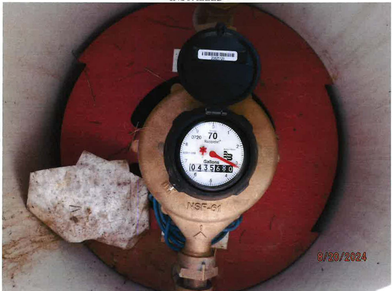
EXAMPLE – SERVICE CONNECTION WITH RECORDALL BRAND FLOWMETER INSTALLED
