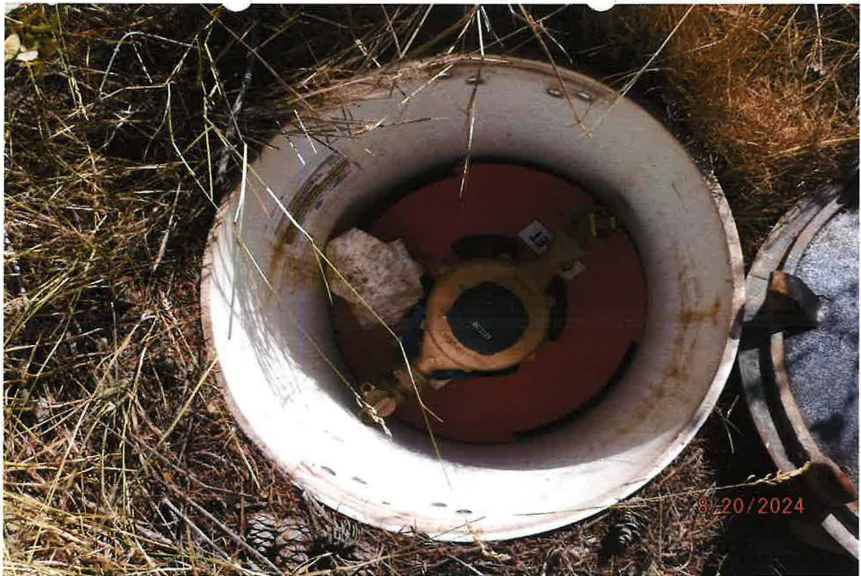
EXAMPLE – SERVICE CONNECTION WITH RECORDALL BRAND FLOWMETER INSTALLED
