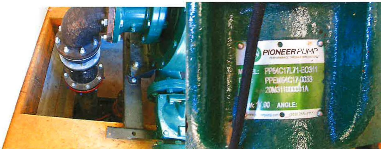
Pump House Equipment , Intake line and Pump Model
