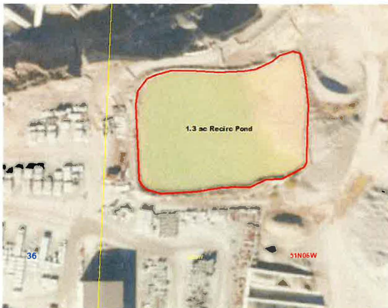
Rock crushing & gravel washing recirculation pond
