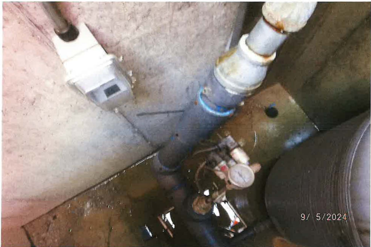
VAULTED WATER CONVEYANCE SYSTEM PRESSURE TANKS 6-EA & DISTRIBUTION PIPELINE TO DOMESTIC USES (CO-LOCATED WITH STORAGE RESERVOIR)
