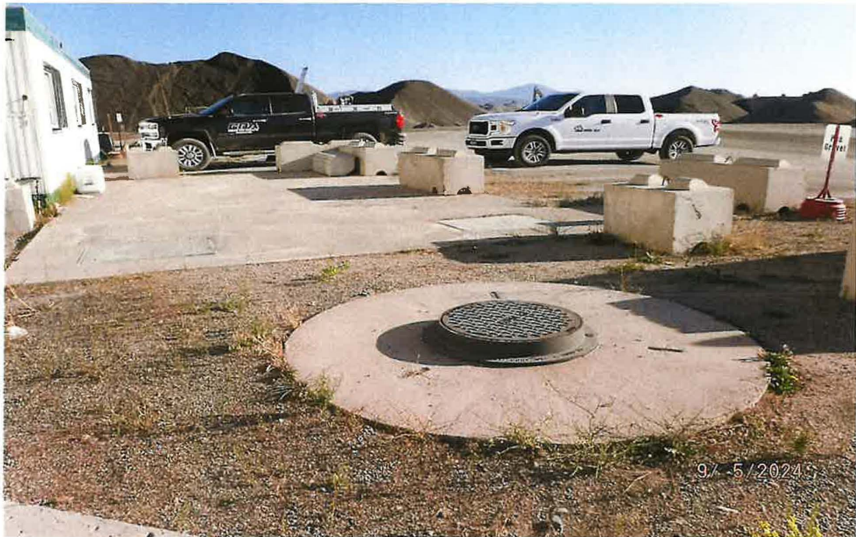
STANDING BETWEEN PUMP STATION CONTROL PANEL TREE & WELL D0069998. 30,000-GAL STORAGE RESERVIOR CONCRETE RECTANGLE IN IMAGE; WELL D0079452 LOCATED BEHIND BLACK TRUCK IN IMAGE
