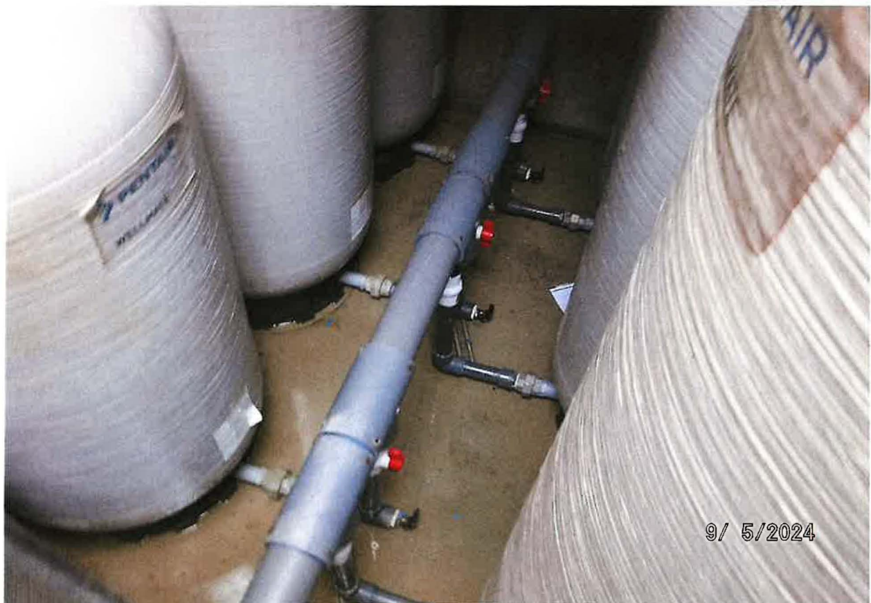
VAULTED WATER CONVEYANCE SYSTEM PRESSURE TANKS 6-EA & DISTRIBUTION PIPELINE TO DOMESTIC USES (CO-LOCATED WITH STORAGE RESERVOIR)
