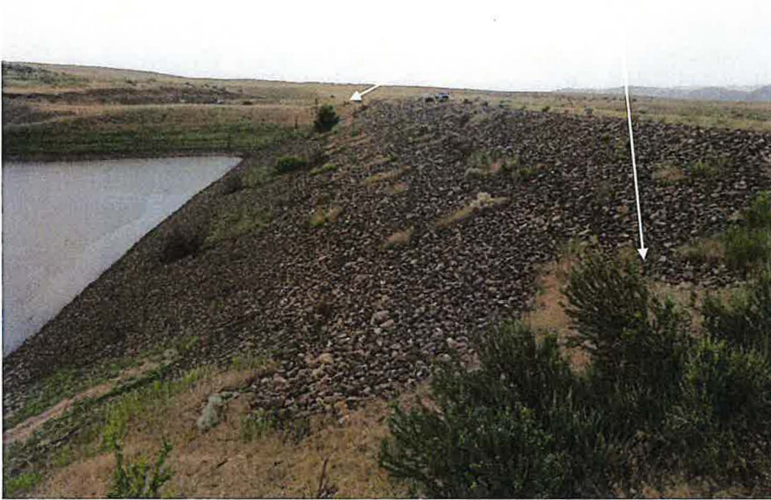
Photo 3: Upstream slope; notice minor amount of woody vegetation
