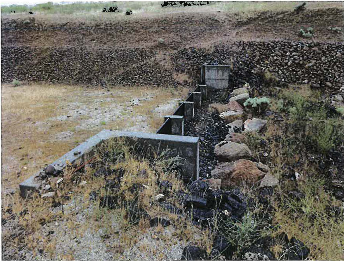
Photo 11: Primary spillway with flashboard controlled entrance.
