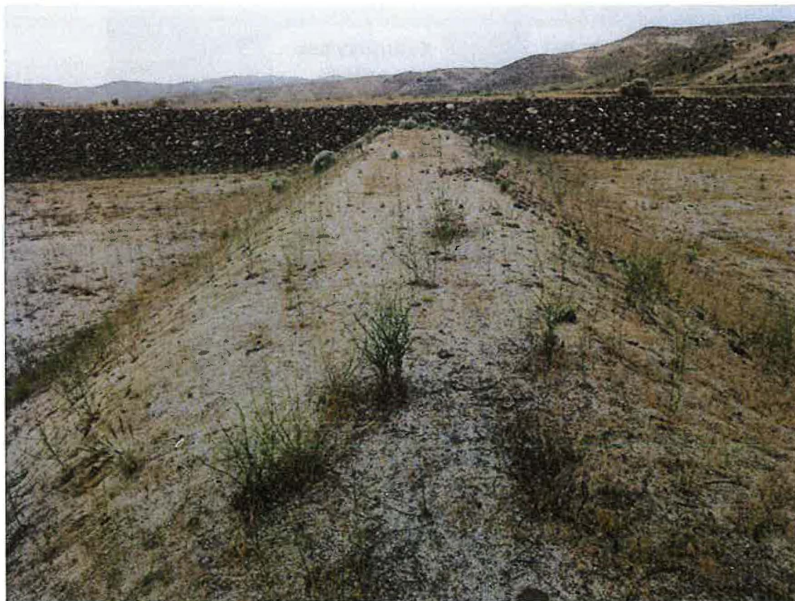
Photo 12: Emergency fuse plug spillway.
