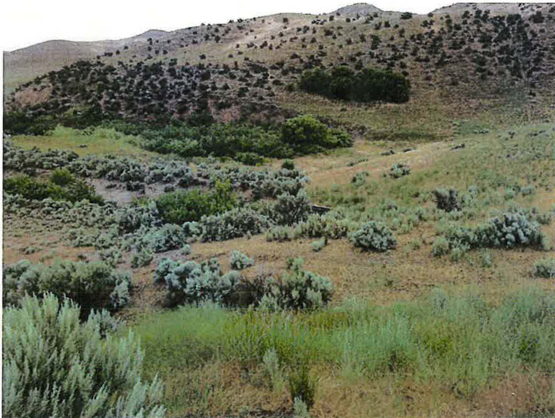
Photo 6: Downstream toe; notice location of outlet.
