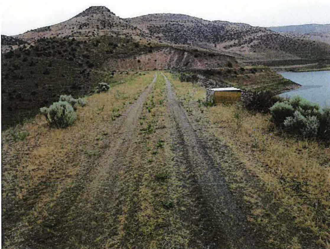
Photo 4: Crest and locked outlet control house; notice minor ruts from vehicles.
