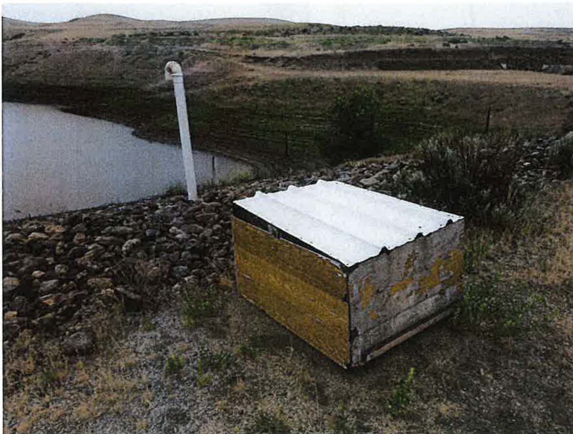
Photo 7: Outlet control house with vent.
