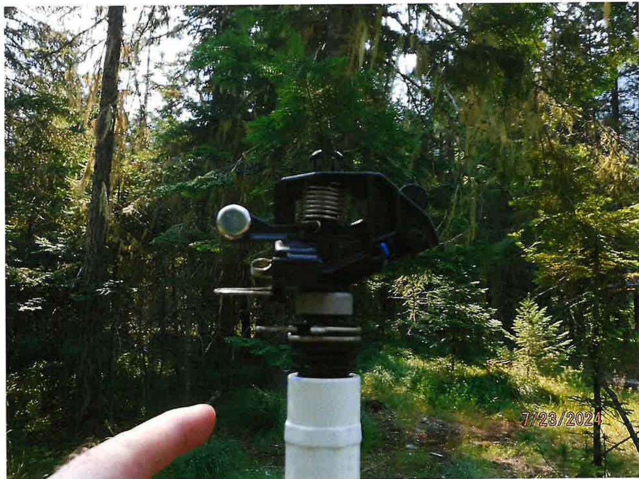
EXAMPLE – IRRIGATION RISER PIPE FROM MAIN SERVICE LINE
