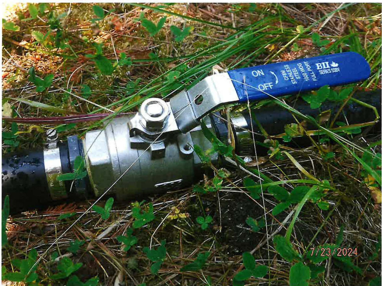
1 1/2 INCH POLYPIPE MAIN IRRIGATION LINE WITH LOCKABLE BALL VALVE INSTALLED NEAR PUMP PRIOR TO DISTRIBUTION TO SPRINKLER SYSTEM
