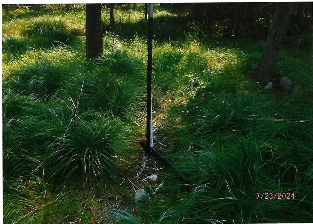
IRRIGATION POU – END OF SYSTEM SPRINKLER ALONG ROADWAY THROUGH PARCEL
