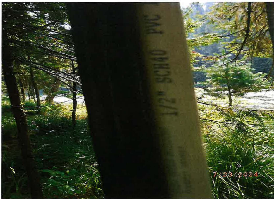
EXAMPLE – ½ INCH RISER PIPE TO IMPACT SPRINKLERS FOR IRRIGATION
