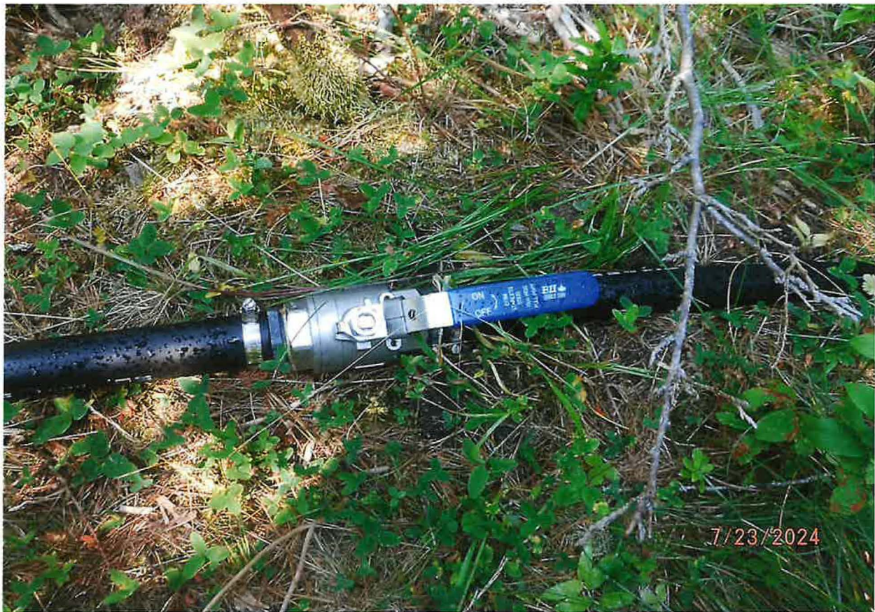
1 1/2 INCH POLYPIPE MAIN IRRIGATION LINE WITH LOCKABLE BALL VALVE INSTALLED NEAR PUMP PRIOR TO DISTRIBUTION TO SPRINKLER SYSTEM
