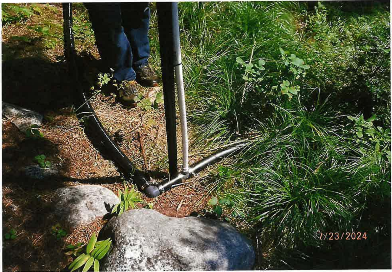
EXAMPLE – IRRIGATION RISER PIPE FROM MAIN SERVICE LINE
