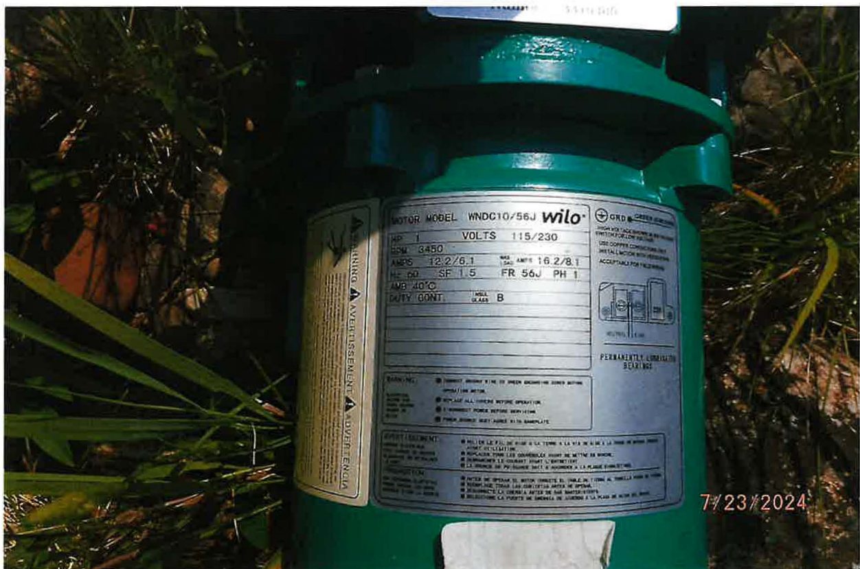
POD – WIL0 BRAND 1 HP ELECTRIC PUMP MOTOR MODEL WND10/56J
