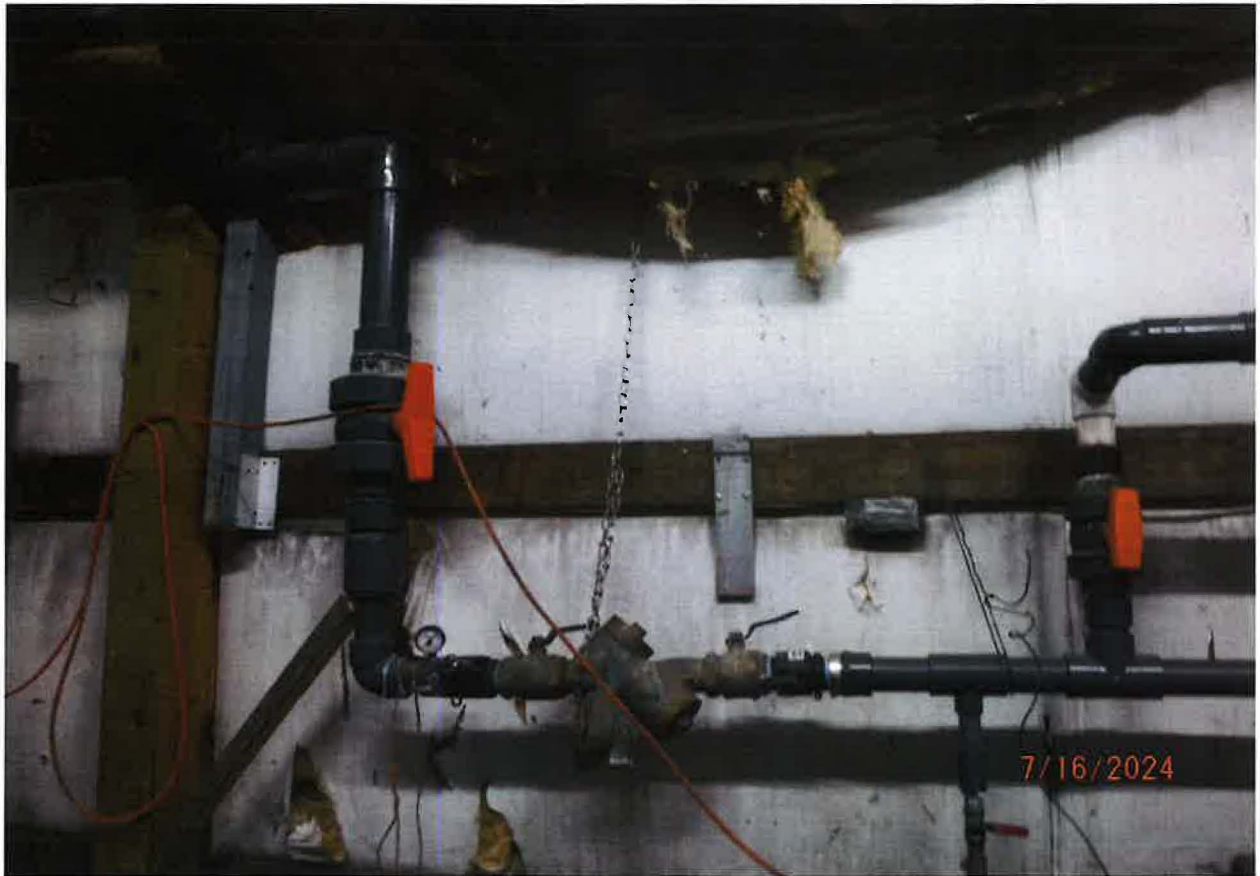
COMMERICAL WATER CONVEYANCE SYSTEM PIPING & FERTILIZER MIXING STATION
