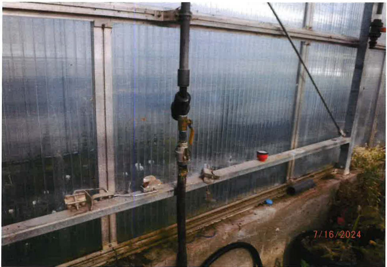
COMMERICAL POU – WATER LINES ROUTE ALONG RAFTERS AND DROP DOWN WITH BANJOY CONNECTIONS TO HOSES AT INTERVALS
