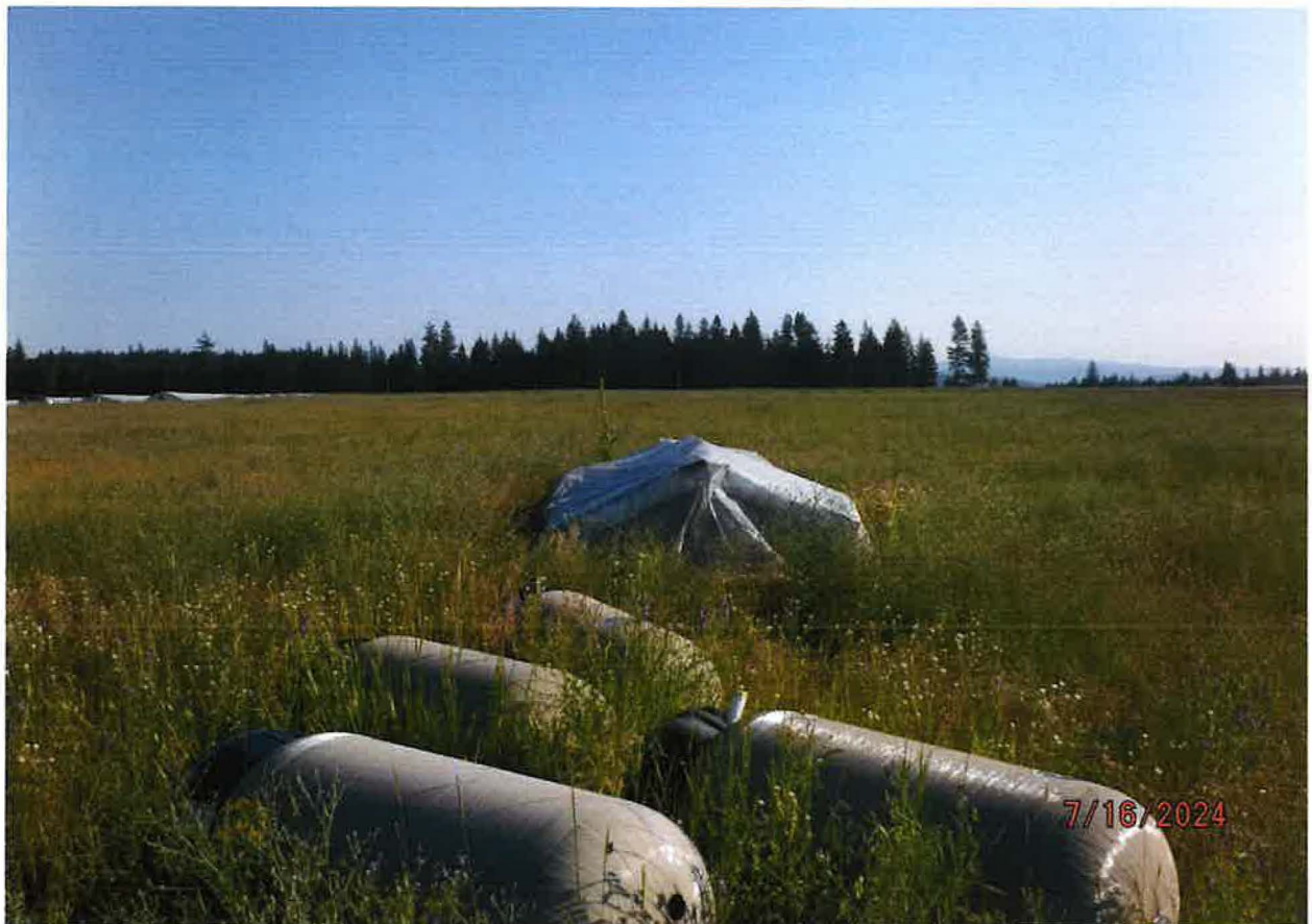
POD – OLD GW WELL IN VAULTED PUMP STATION; STRUCTURE COVERED BY PLASTIC IN PHOTOGRAPH
