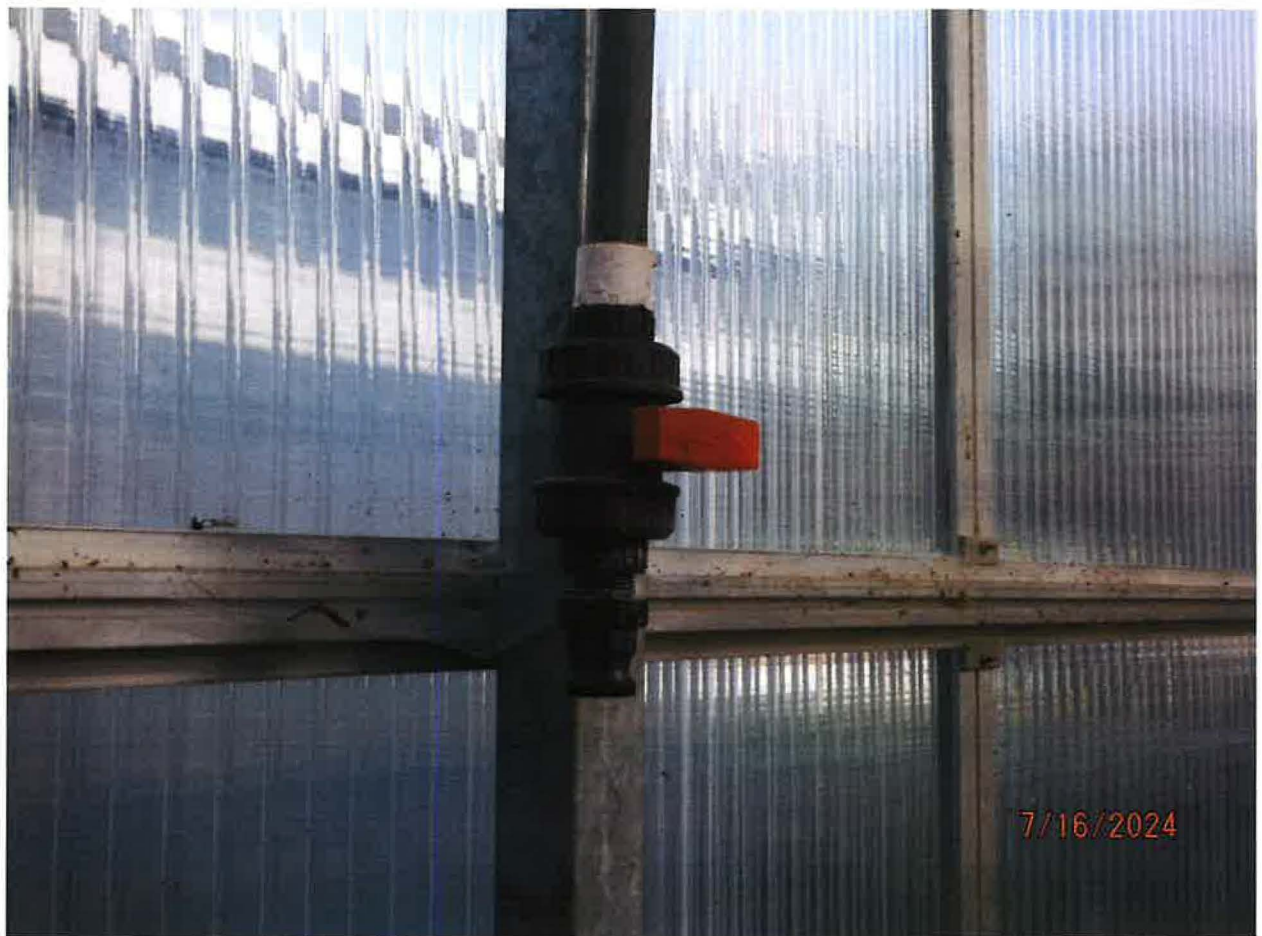
COMMERICAL POU – WATER LINES ROUTE ALONG RAFTERS AND DROP DOWN WITH BANJOY CONNECTIONS TO HOSES AT INTERVALS
