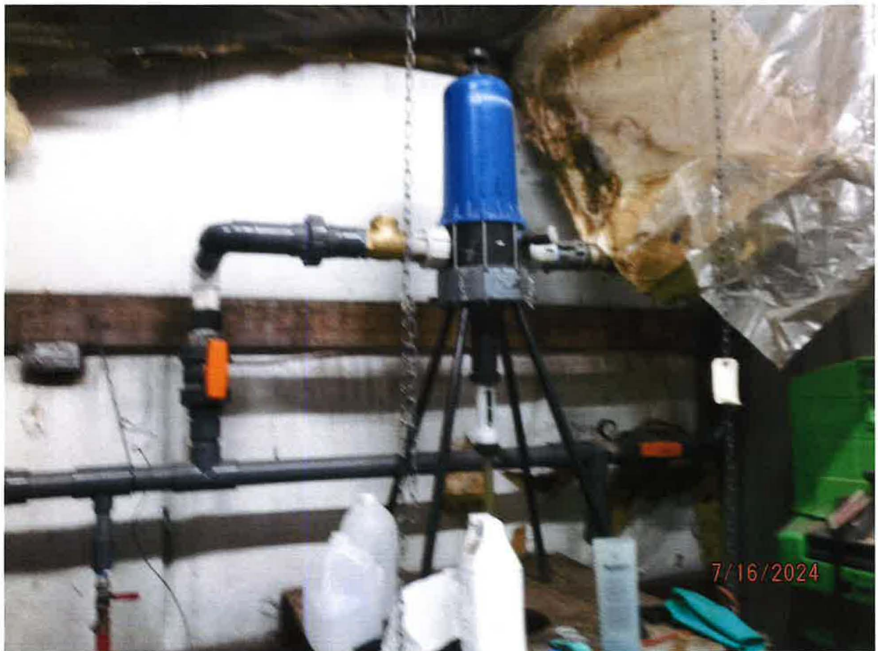
COMMERICAL WATER CONVEYANCE SYSTEM PIPING & FERTILIZER MIXING STATION
