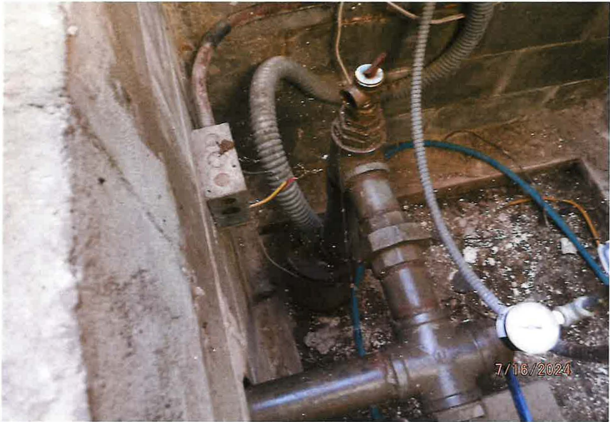
GROUNDWATER WELL – NOT DOCUMENTED IN DEPARTMENT WELL CONSTRUCTION DATABASE
