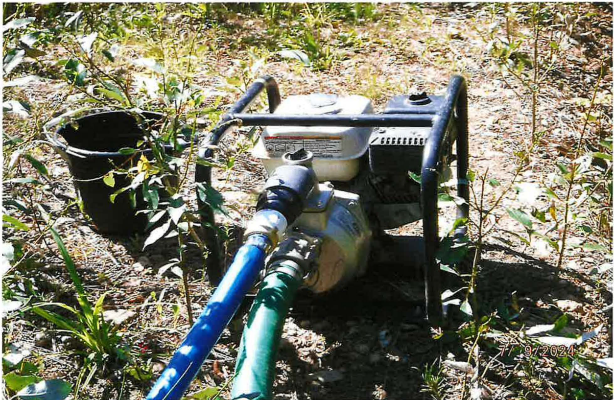
2-INCH OVERFLOW DISCHARGE PORT NECKED DOWN TO FLEXIBLE 1 ½ INCH BLUE FIRE HOSE (100 FT X 2 HOSES) CONNECTED TO BIG GUN SPRINKLER FOR IRRIGATION
