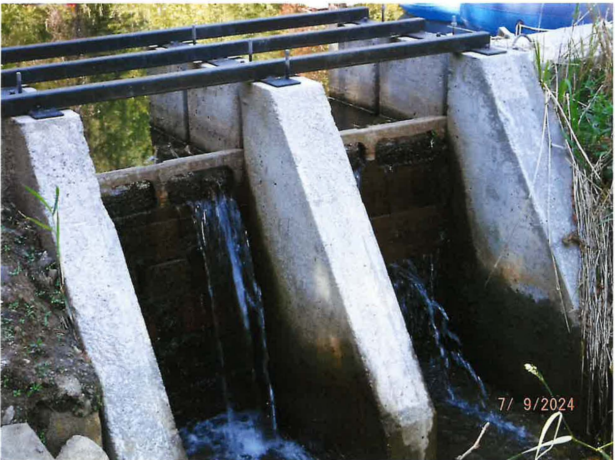
24-HR IMPOUNDMENT POND – CONSTRUCTED IN-STREAM WITH CONCRETE HEADGATE USING WOODEN PLANK INSERTS
