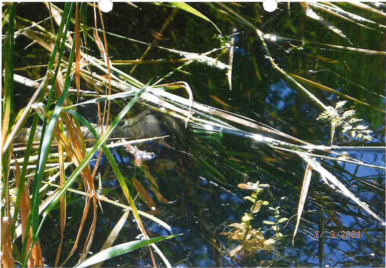
POD – UPPER 24-HR IMPOUNDMENT POOL SCREENED INTAKE TO WATER TRANSFER PUMP
