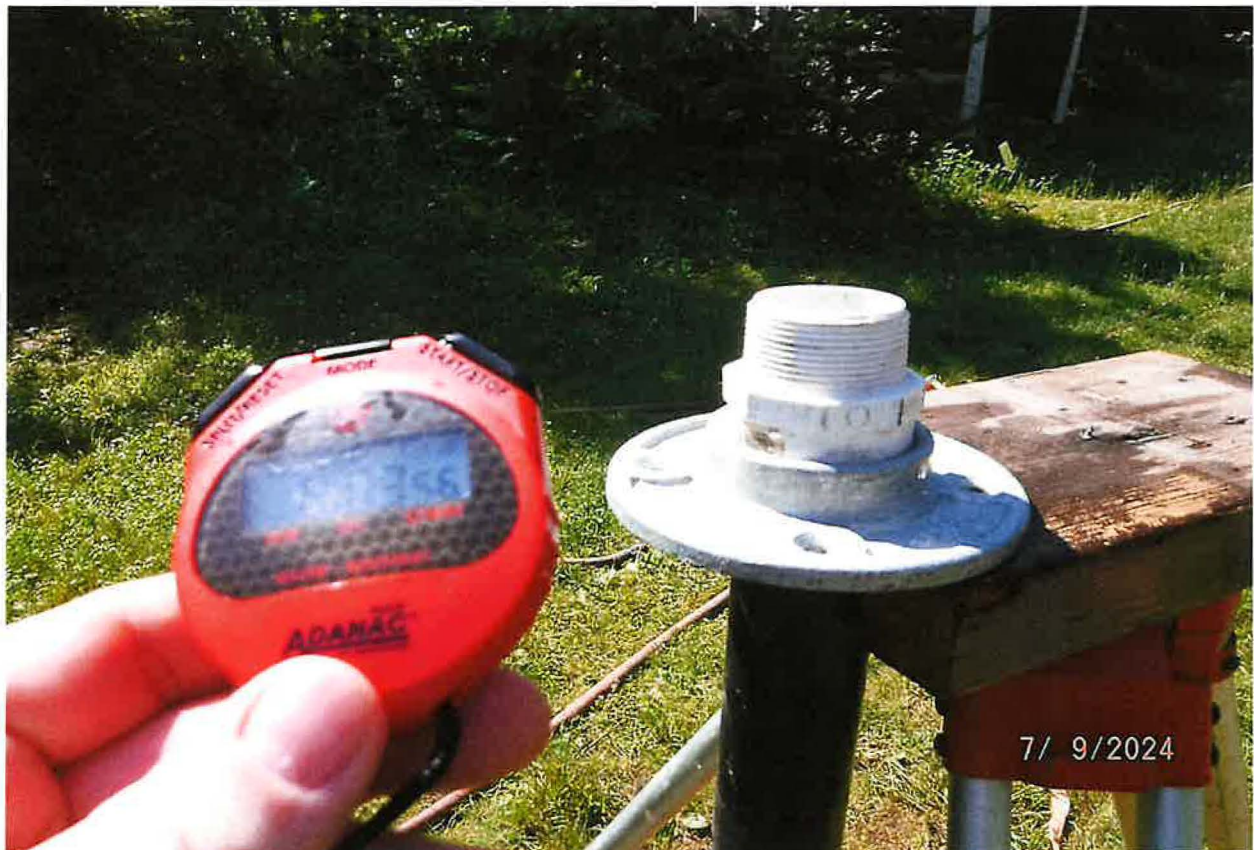
5-GAL BUCKET MEASUREMENT ATTEMPTED FROM 1-1/2 INCH IRRIGATION RISER PIPE AT SPRINKLER ATTACHMENT – UNABLE TO USE MEASUREMENT DUE TO FILE TIME REQUIREMENTS (< 5 SECONDS)
