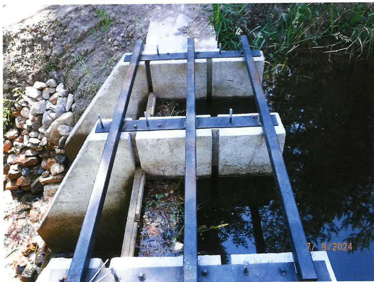
24-HR IMPOUNDMENT POND – INSTREAM WITH HEADGATE CONSTRUCTION
