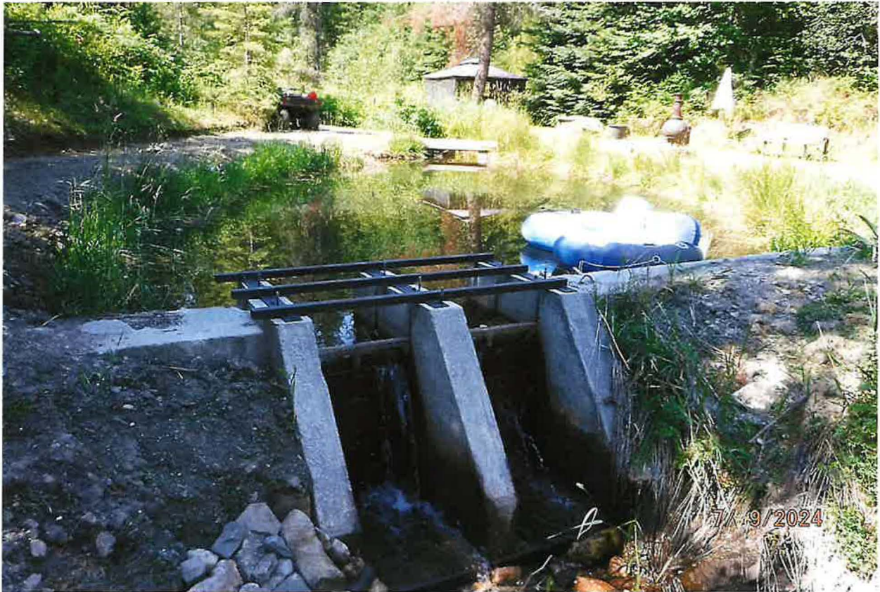
24-HR IMPOUNDMENT POND – CONSTRUCTED IN-STREAM WITH CONCRETE HEADGATE USING WOODEN PLANK INSERTS
