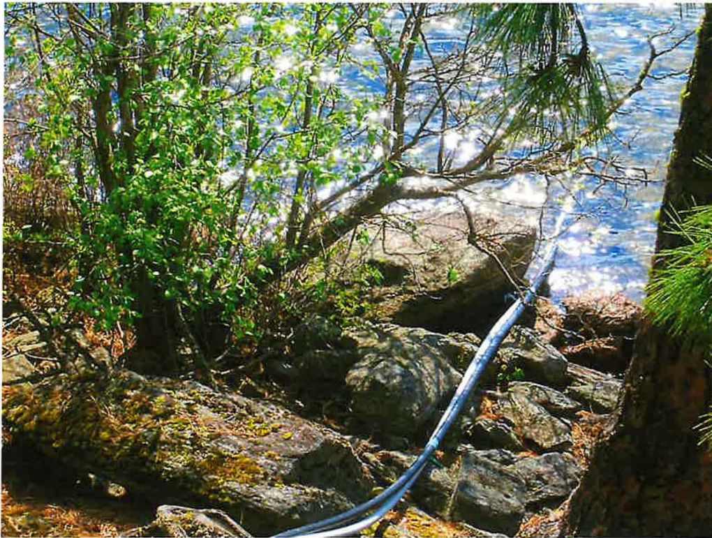
Intake Lines with lift uphill to pump house
