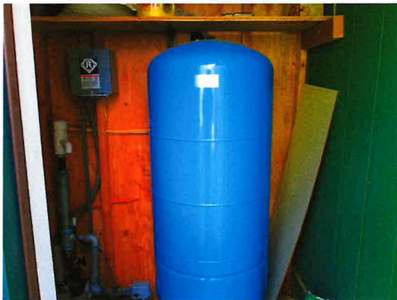
Continued Lift to red pump house with pressure tank inside
