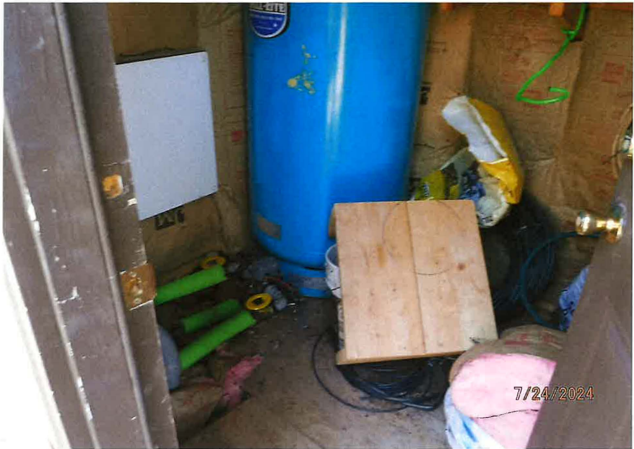
WATER CONVEYANCE SYSTEM INCORPORATES WELL PUMPING DIRECTLY TO A PRESSURE TANK BEFORE DISTRIBUTION TO WATER USES
