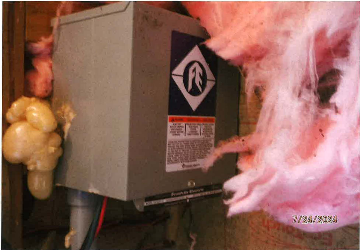
DIVERTING WORKS – 1.5 HP FRANKLIN ELECTRIC PUMP MOTOR MODEL No. 2823008110
