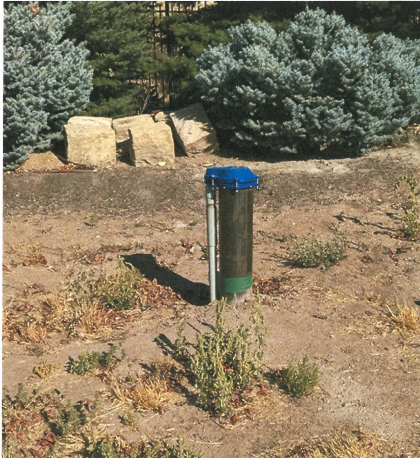
Figure 2 Photo of point of diversion (well head)
