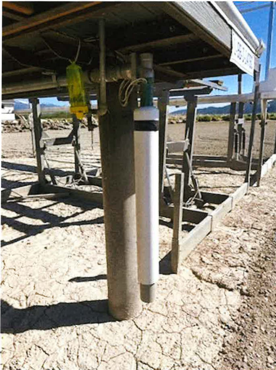
PUMP AND PIPELINE AFFIXED TO DOCK
