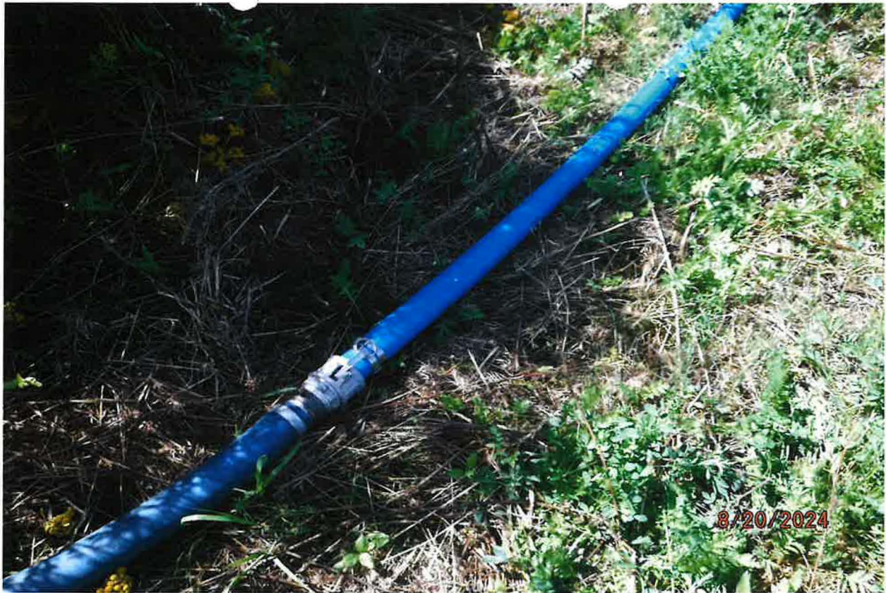
IRRIGATION WATER CONVEYANCE SYSTEM – 2-INCH FLEX FIRE HOSE ROUTED TO 2-INCH ALUMINUM HAND LINE W/IMPACT SPRINKLERS & A SEPARATE BIG GUN SPRINKLER
