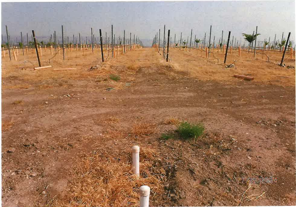
IRRIGATION POU – WATER MAIN LINE TO VINEYARD DRIP IRRIGATION ROW CROPS
