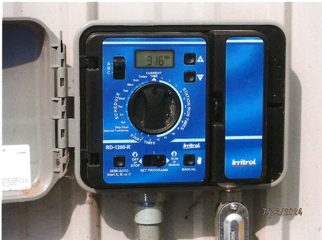
IRRITROL RAIN DIAL IRRIGATION SYSTEM CONTROLLER
