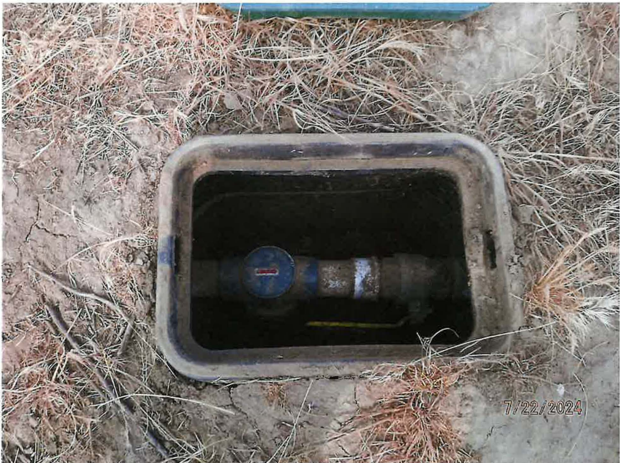
CONVEYANCE FROM PUMP HOUSE TO IRRIGATION POU – MAIN WATER LINE SHUTOFF BOX
