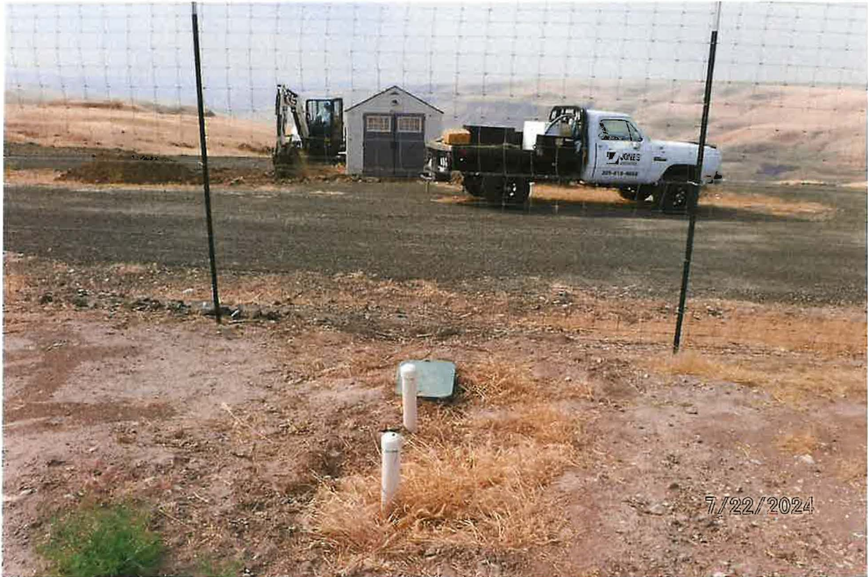
CONVEYANCE FROM PUMP HOUSE TO IRRIGATION POU – MAIN WATER LINE SHUTOFF BOX
