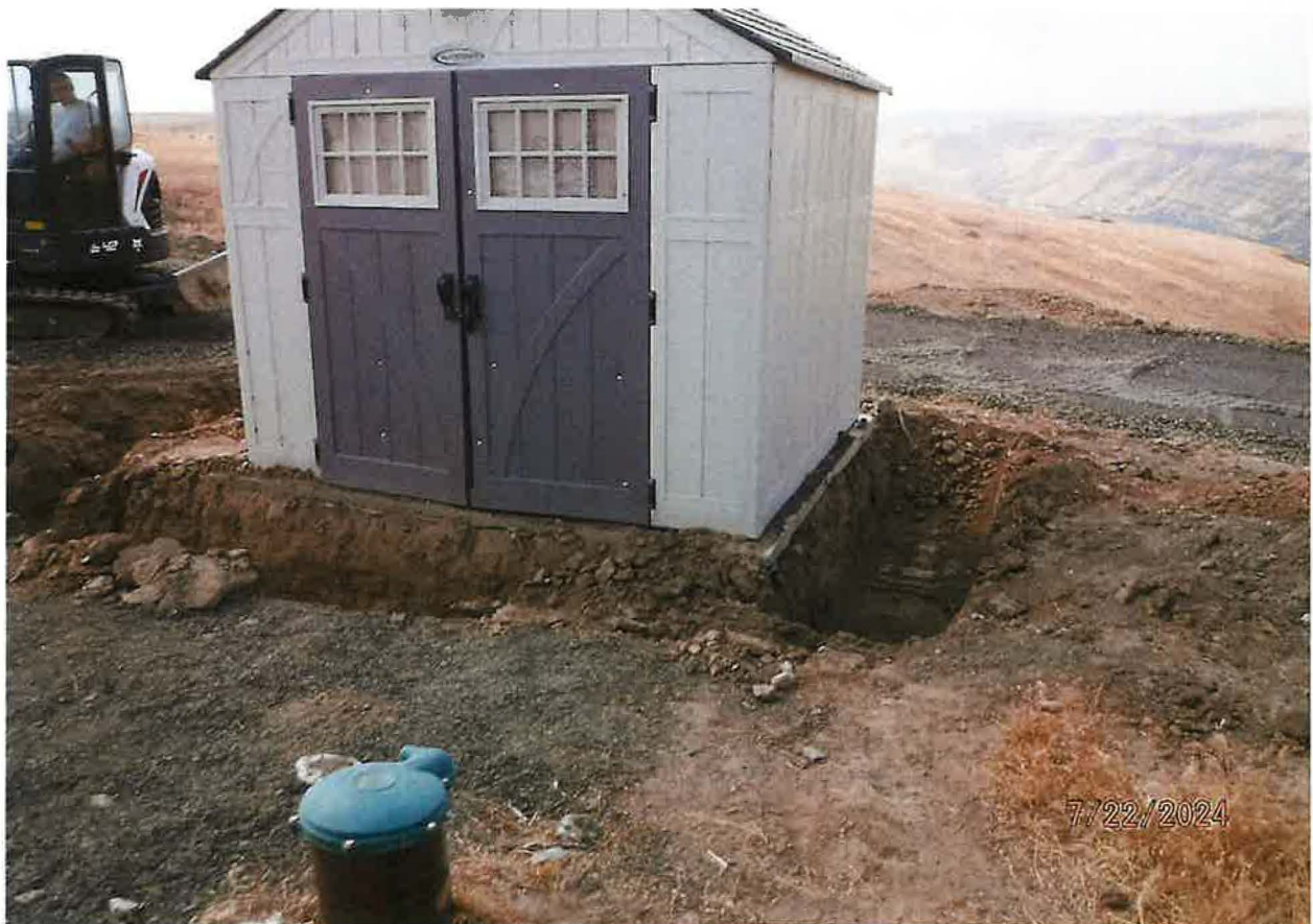
WELL AND PUMP HOUSE
