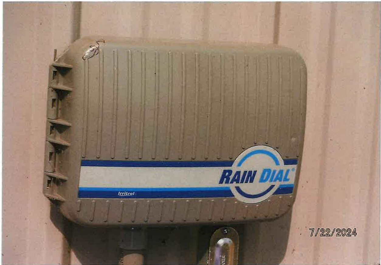
IRRITROL RAIN DIAL IRRIGATION SYSTEM CONTROLLER
