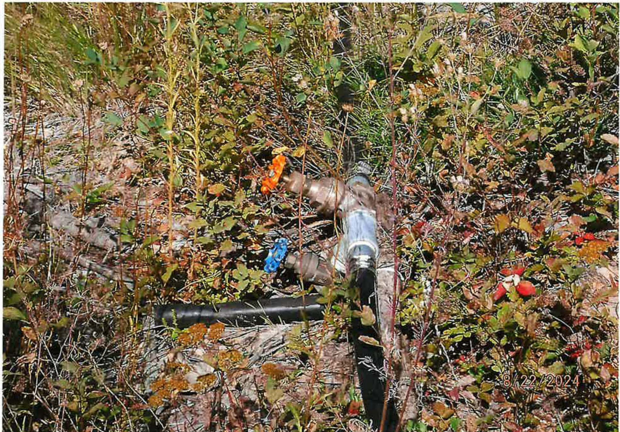
3 RD PRIMER/BLOWOUT VALVE INSTALLED ON MAIN SERVICE PIPELINE
