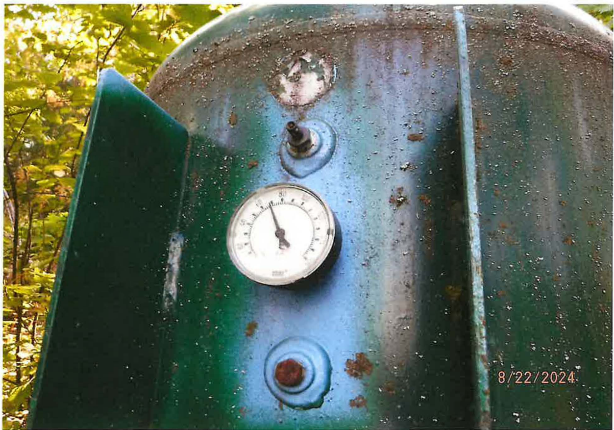
70 PSI WATER SYSTEM STATIC PRESSURE
