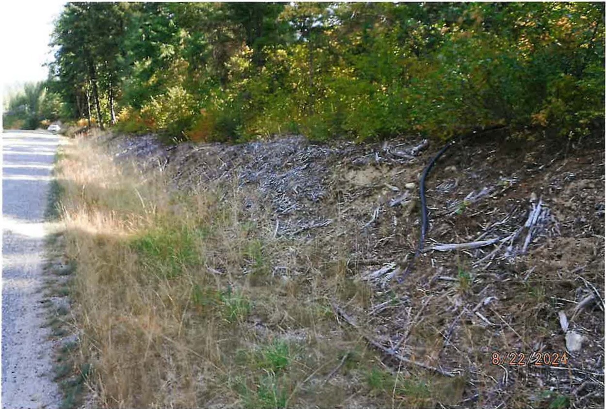
WATER CONVEYANCE PIPELINE ROUTES ABOVE GROUND TO PAVED ROADWAY, THEN GOES UNDER THE ROAD AND DAYLIGHTS WITHIN THE POU
