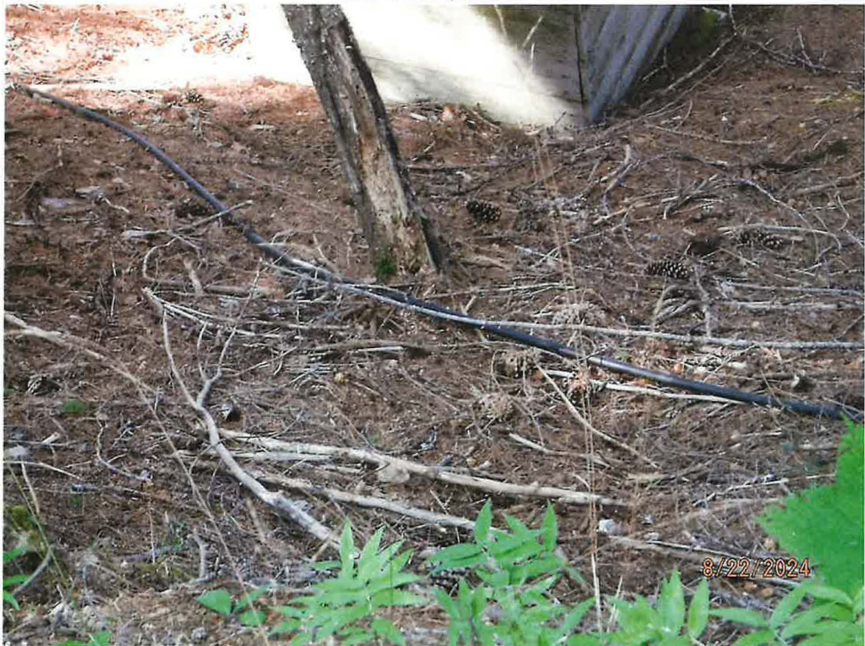
WATER LINE ROUTED ACROSS PARCEL
