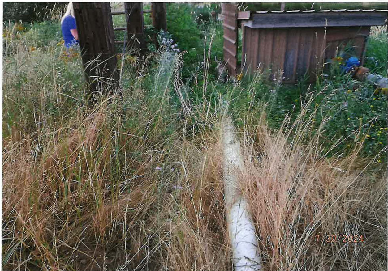
6-INCH ALUMINUM TRANSITIONS TO PVC PIPE CROSSING ROAD AND ROUTING TO 24-HR IMPOUNDMENT POND
