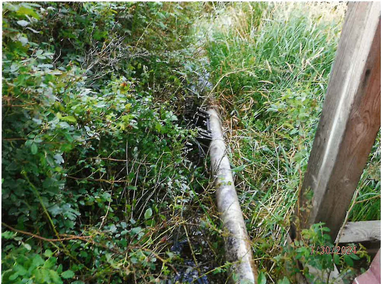
WATER CONVEYANCE PIPE NECKS DOWN TO 4 INCH ALUMINUM WHERE IT DISCHARGES INTO 24-HR IMPOUNDMENT POND
