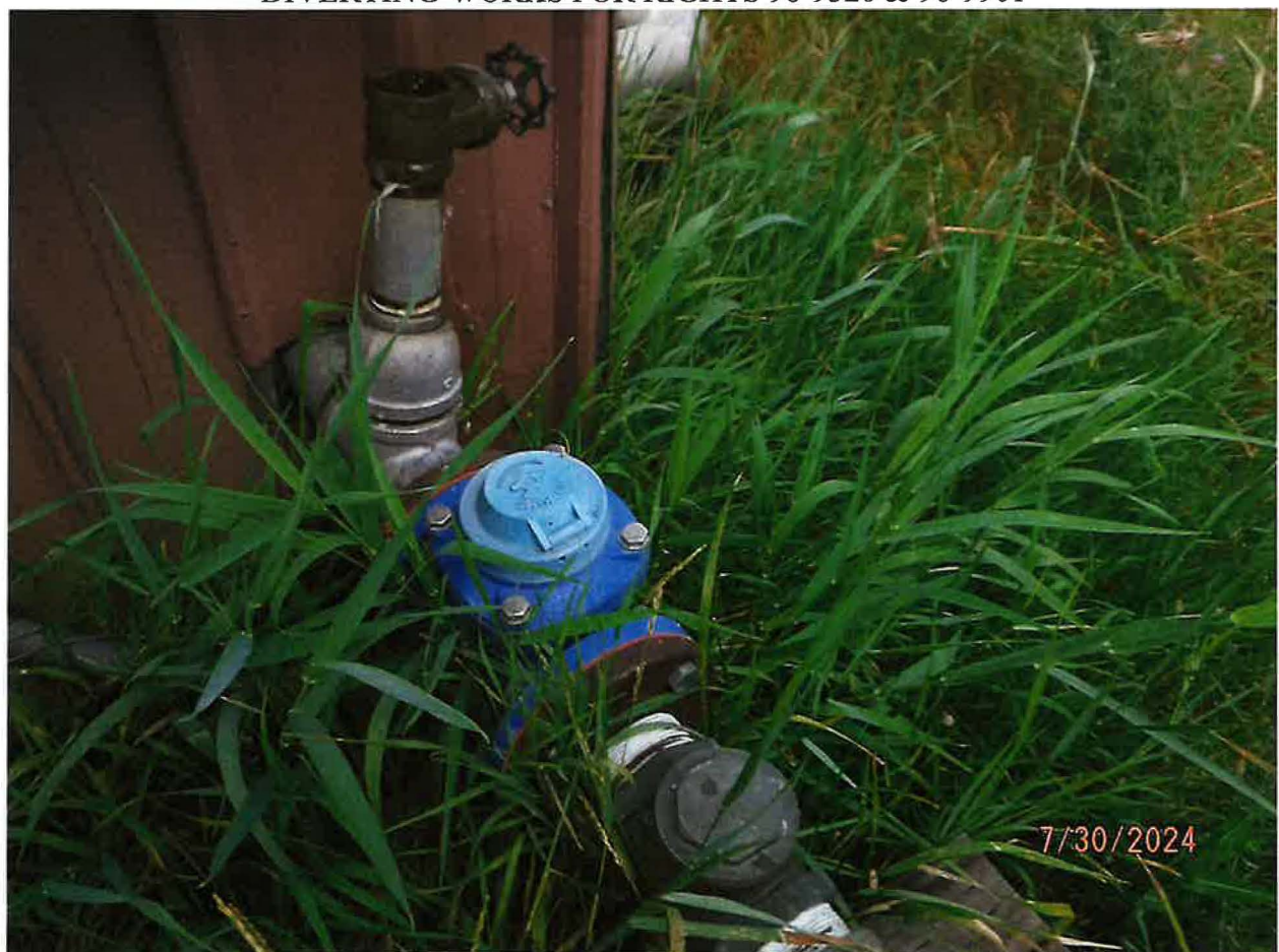
POD – 30 HP CENTRIFUGAL PUMP AND FLOWMETER INSTALLED ON COMMON DIVERTING WORKS FOR RIGHTS 96-9320 & 96-9901
