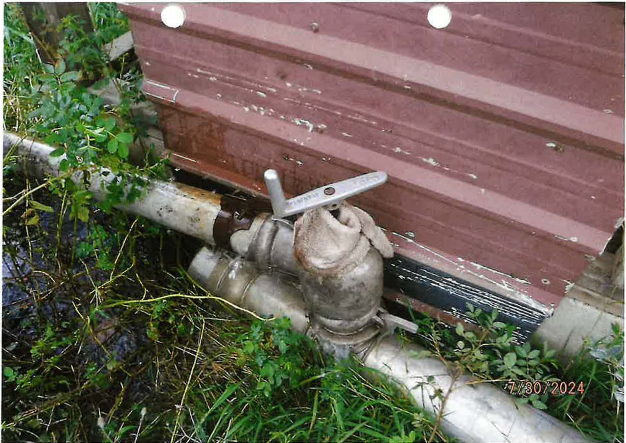
WATER CONVEYANCE PIPE NECKS DOWN TO 4 INCH ALUMINUM WHERE IT DISCHARGES INTO 24-HR IMPOUNDMENT POND
