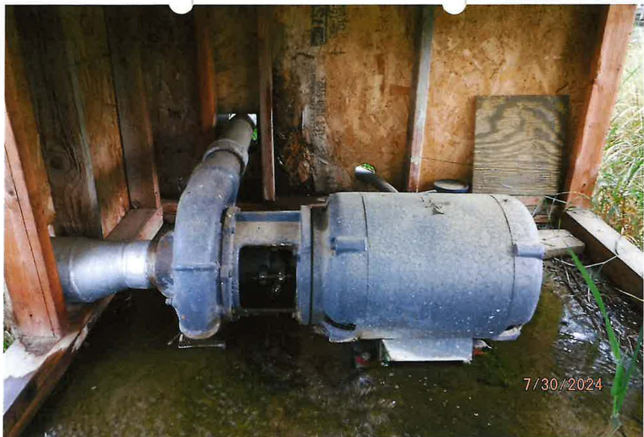
POD – 30 HP CENTRIFUGAL PUMP AND FLOWMETER INSTALLED ON COMMON DIVERTING WORKS FOR RIGHTS 96-9320 & 96-9901
