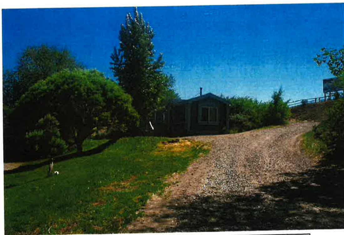
Heated Residence Near SE Corner of Campground Looking East By J E Stanton 6-5-2002
