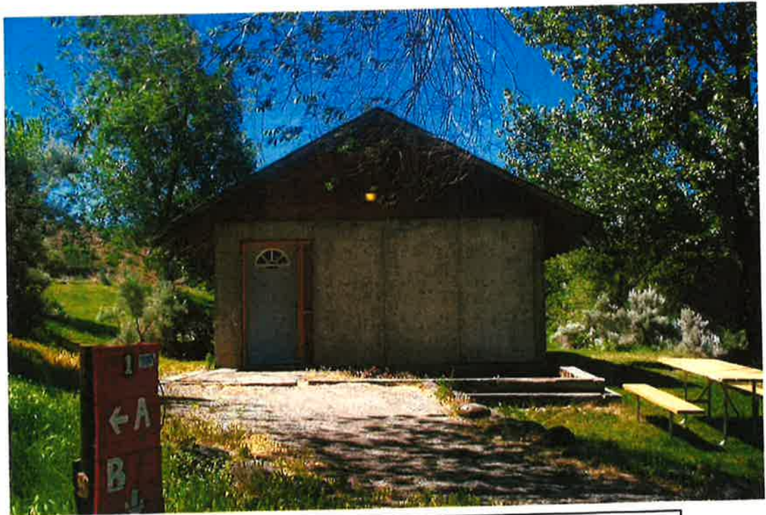
Heated Restroom At Campground NE of Hot Well Looking West By J E Stanton 6-5-2002
