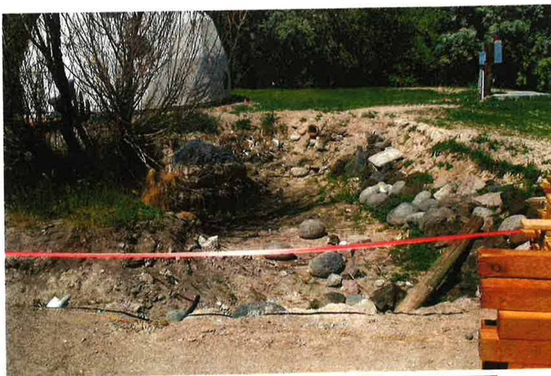
Alligator Pond South of Hot Well Looking South West (Currently Undergoing Reconstruction) By J E Stanton 6-5-2002
