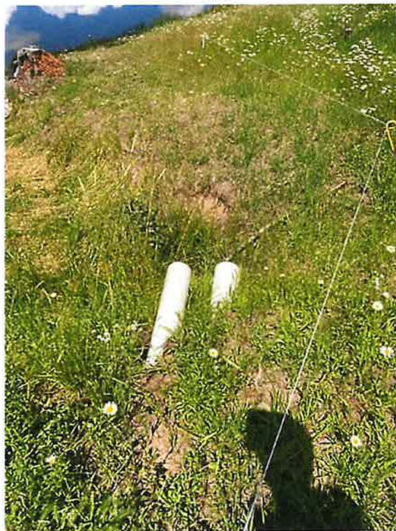
Figure 6: Overflow from the upper pond to the lower pond, facing north
