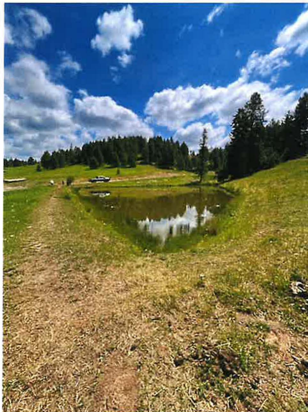
Figure 4: Downstream Pond facing southeast. Embankment runs towards truck along north edge of pond. Notice livestock dung
