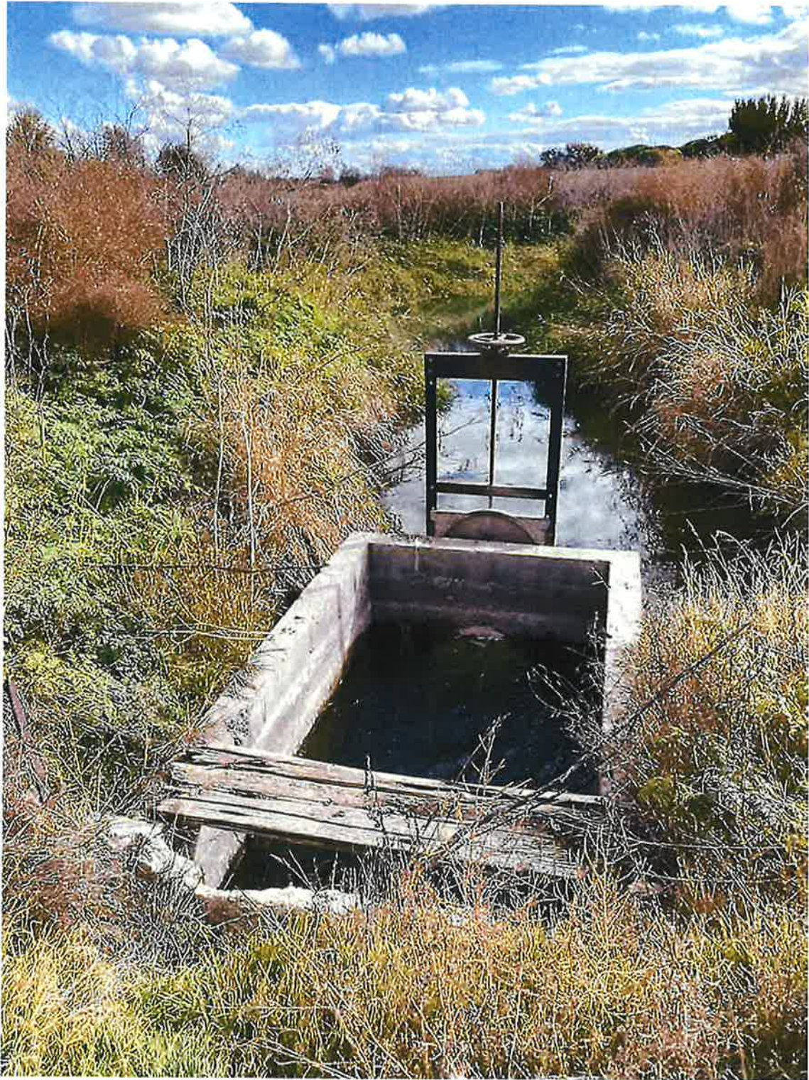
Lockable headgate at point of diversion.
