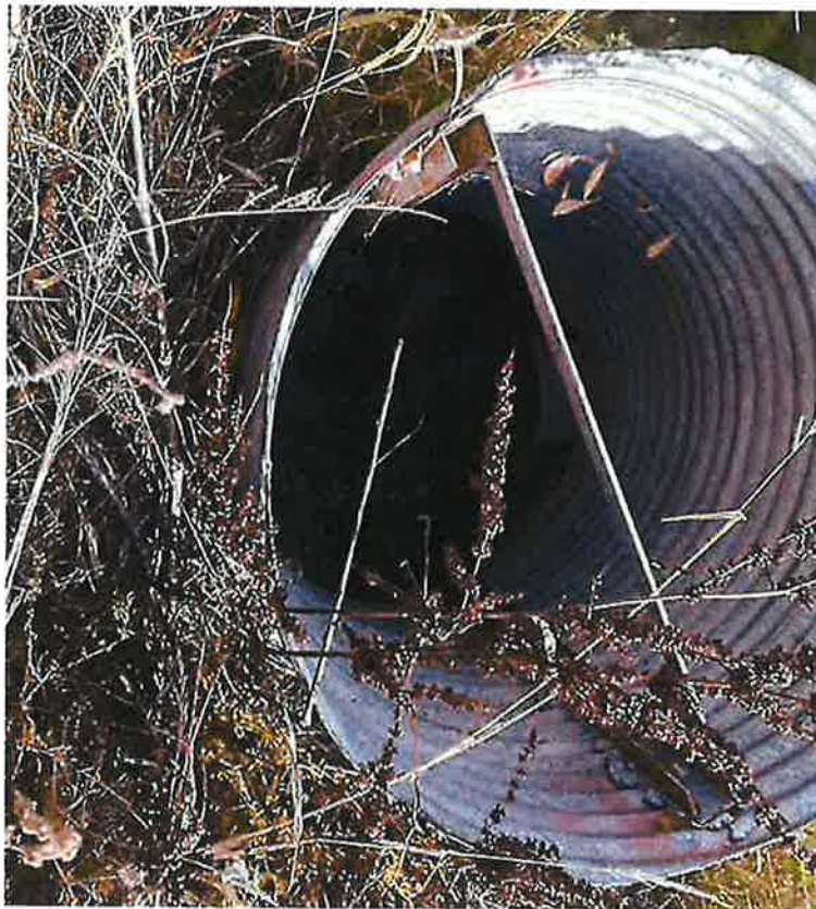
Outlet structure at Beaver Pond
