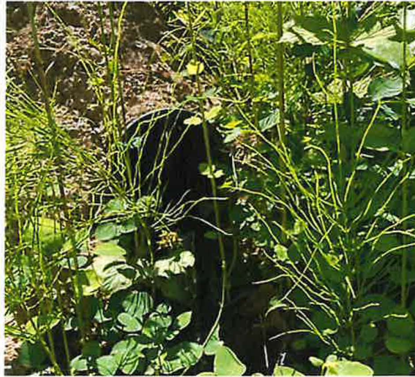
Figure 5: Culvert from which measurement was taken
