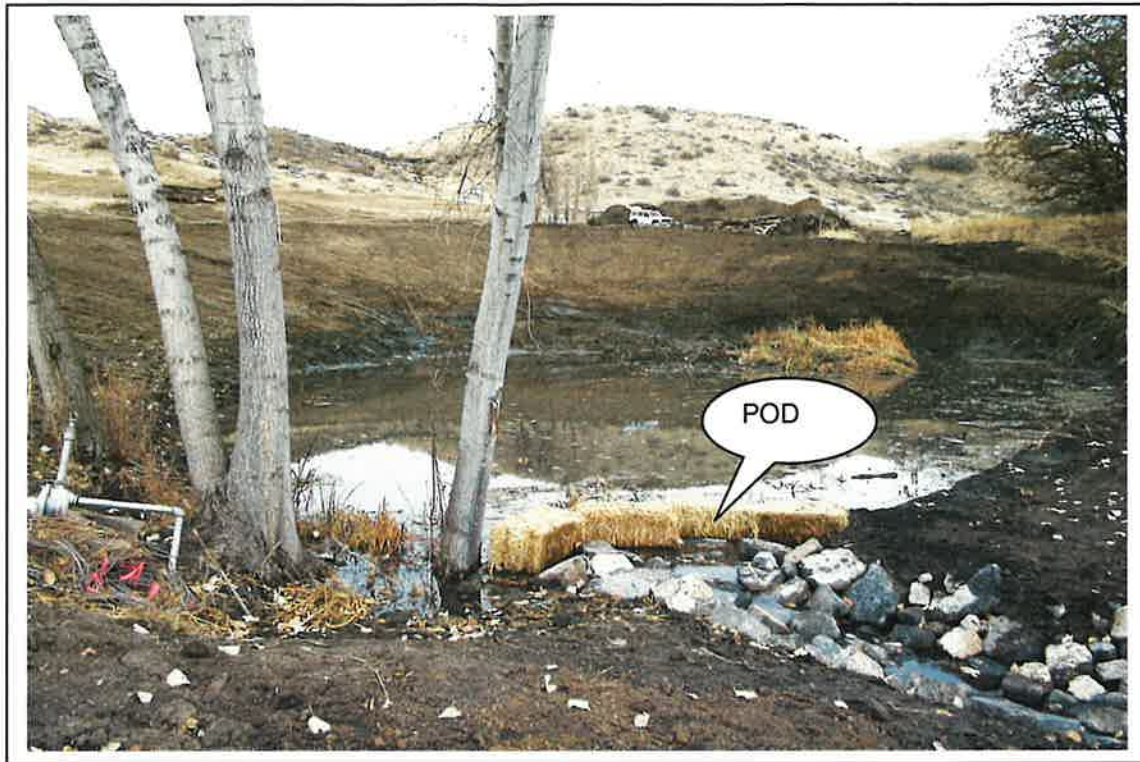
Photo 1: 63-31586, Field Exam 11-15-02: Spring in pond. Earth, rock, straw dam. The POD is located in the SESWNW, S29, T05N, R02E. Pond is approximately 5' deep and has a surface area of 0.2 acres per GIS. Fire protection storage is 0.40 AF. See attached maps. Enlargement of right 63-31247.
