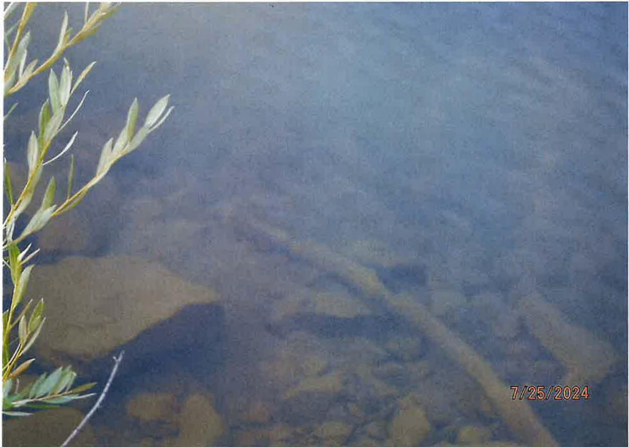
POD – SCREENED INTAKE IN COEUR D'ALENE RIVER
