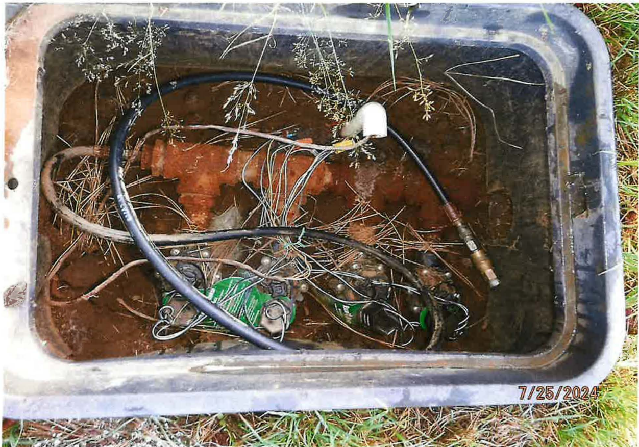
WATER CONVEYANCE SYSTEM USES FOUR ZONES FOR DOMESTIC EXTERNAL USE UP TO ½ ACRE IRRIGATION BY PRESSURIZED SPRINKLERS
