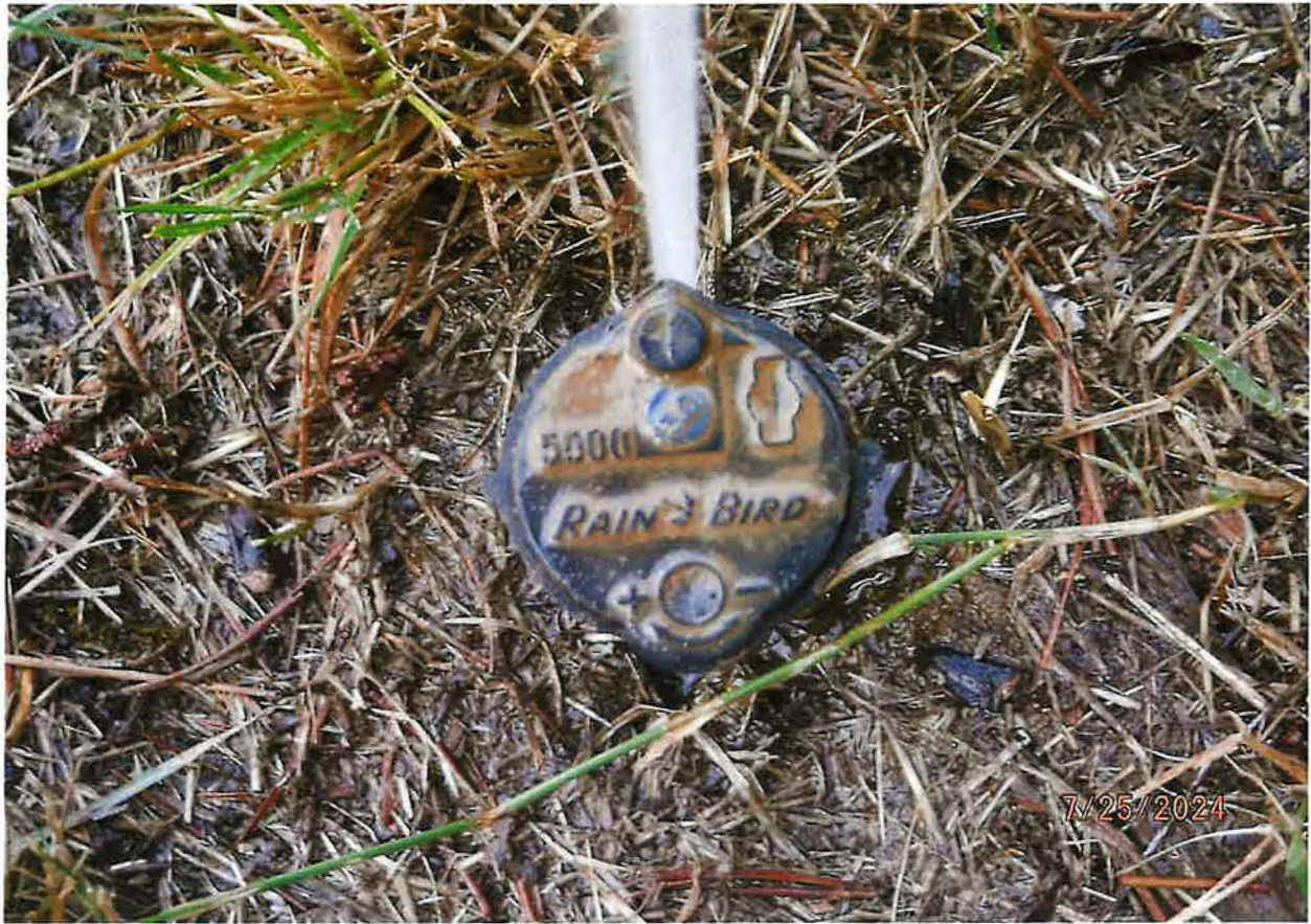
DOMESTIC POU – EXTERNAL USE ONLY, ½ ACRE IRRIGATION USES RAIN BIRD 5000 POP-UP ROTARY SPRINKLERS TO IRRIGATE RIVER FRONTAGE AT THE POU
