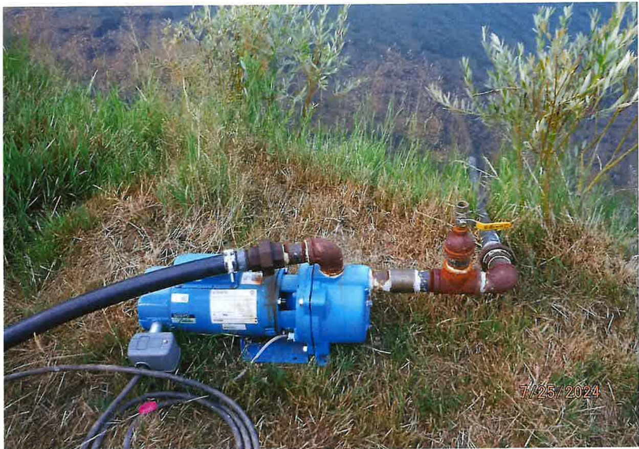
POD – 1.5 HP U.S. MOTORS CENTRPRO CENTRIFUGAL PUMP TO 1.5-INCH DISCHARGE PIPELINE
