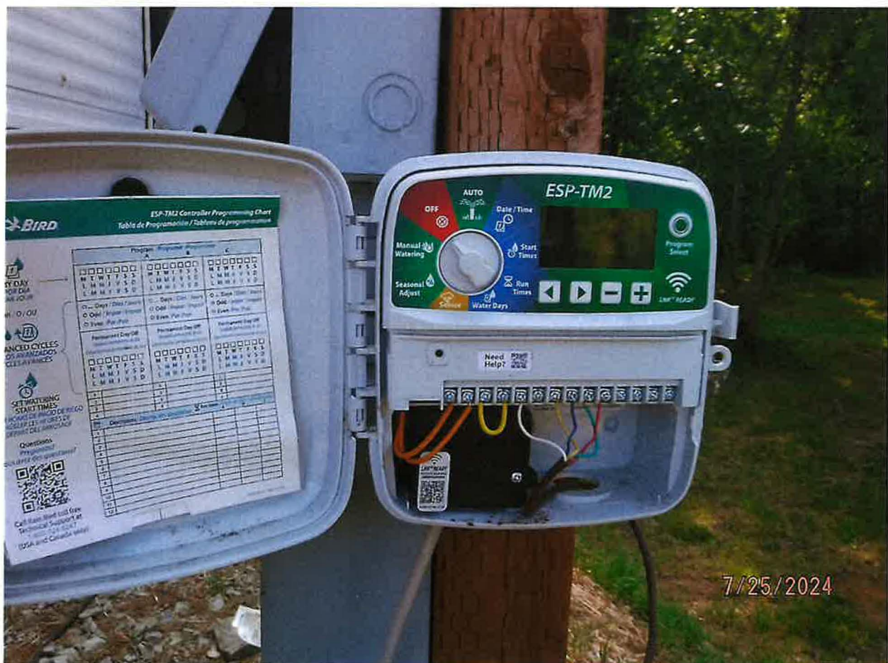
WATER CONVEYANCE SYSTEM USES FOUR ZONES FOR DOMESTIC EXTERNAL USE UP TO ½ ACRE IRRIGATION BY PRESSURIZED SPRINKLERS
