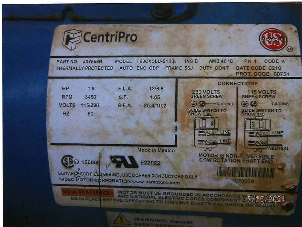
POD – 1.5 HP U.S. MOTORS CENTRPRO CENTRIFUGAL PUMP TO 1.5-INCH DISCHARGE PIPELINE
