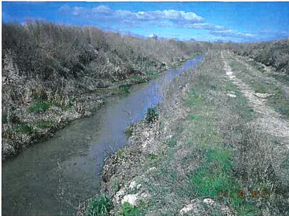
Photo 4: Haas Canal looking downstream
