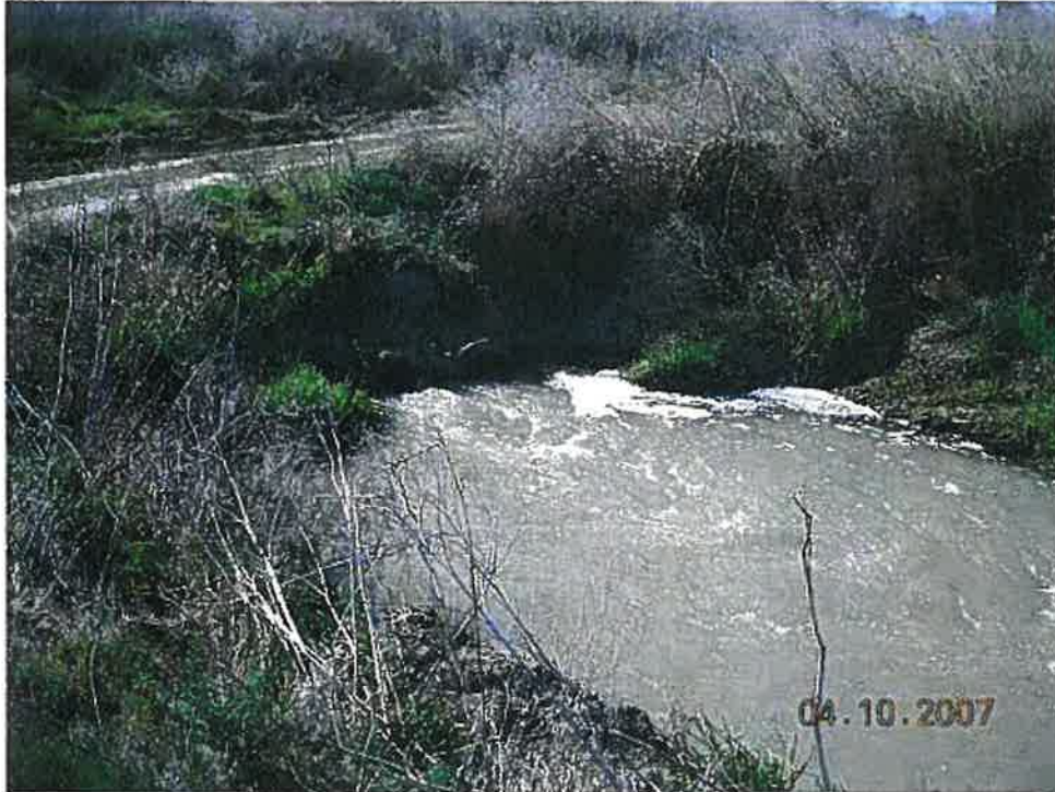
Photo 3: Discharge from the 24-inch Headgates into the Haas Canal
