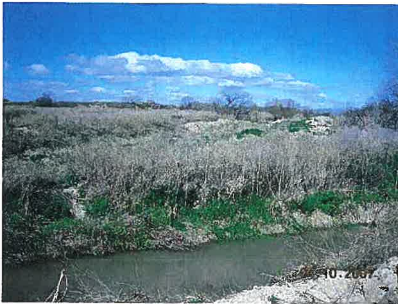
Photo 5: Location of Proposed Headgate to take Water from Haas Canal (foreground) to the East End Drain (center of picture).
