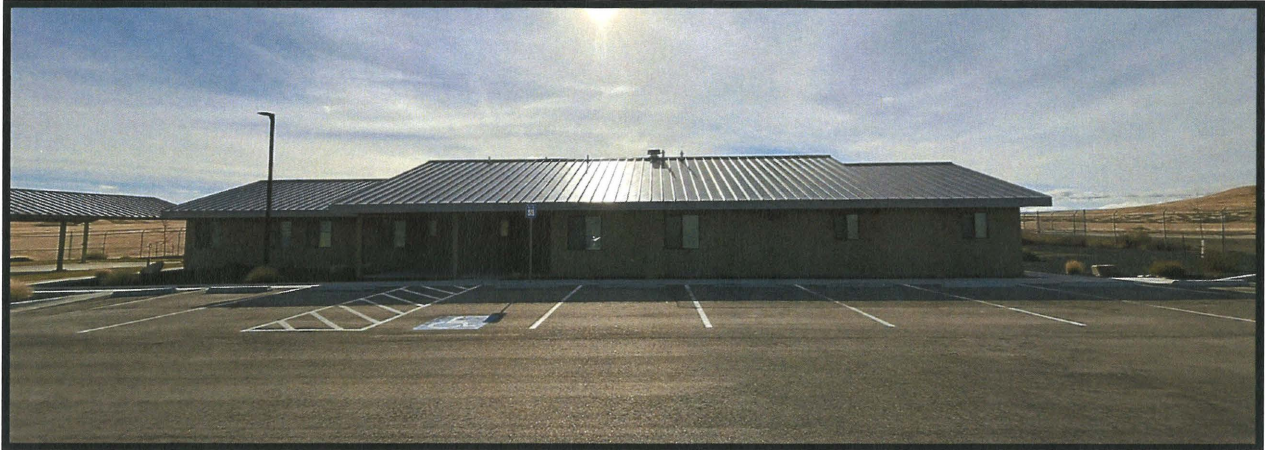
Photo 7- (facing south) The crew quarters building north of the pump house with the common area visible to the east (left).
