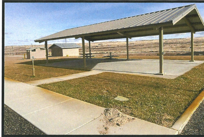
Photo 4- Irrigated common area facing NE control valve and drain box in the foreground. One of the frost free spigots is seen near the leading to the gazebo area.
