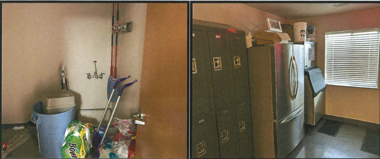
Photo 14 & 15- (above) Locker room in the crew quarters building includes a mop sink, refrigerator with water hook up, and ice machine.
