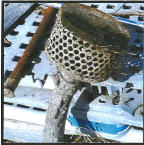
Photo 3- 1/4" Fish screen on poly intake line.
