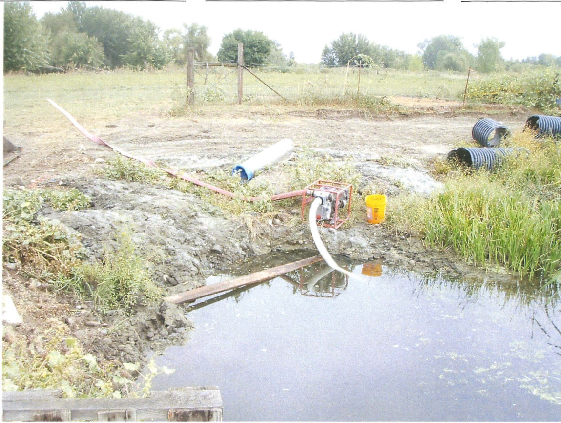
Figure 1. Diversion point 1 with 3-inch trash pump from unnamed drain to pasture.
