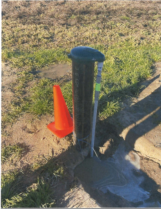
Figure 3 Well head D0104334 located at 44.02751 -116.91985.
