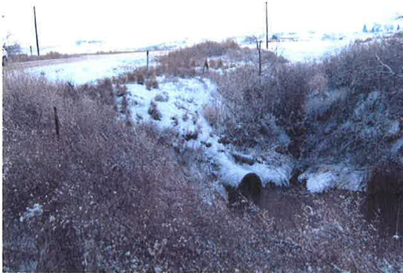
Photo 1: Hwy 95 Culvert for Baldridge and Meadows Drain T5N R5W S27 NESE (facing south)
