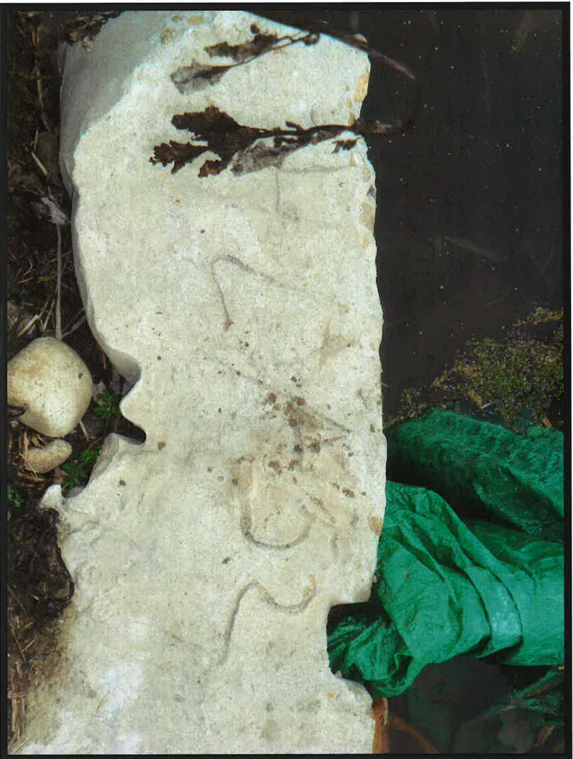
7B. 1952 Diversion Structure
