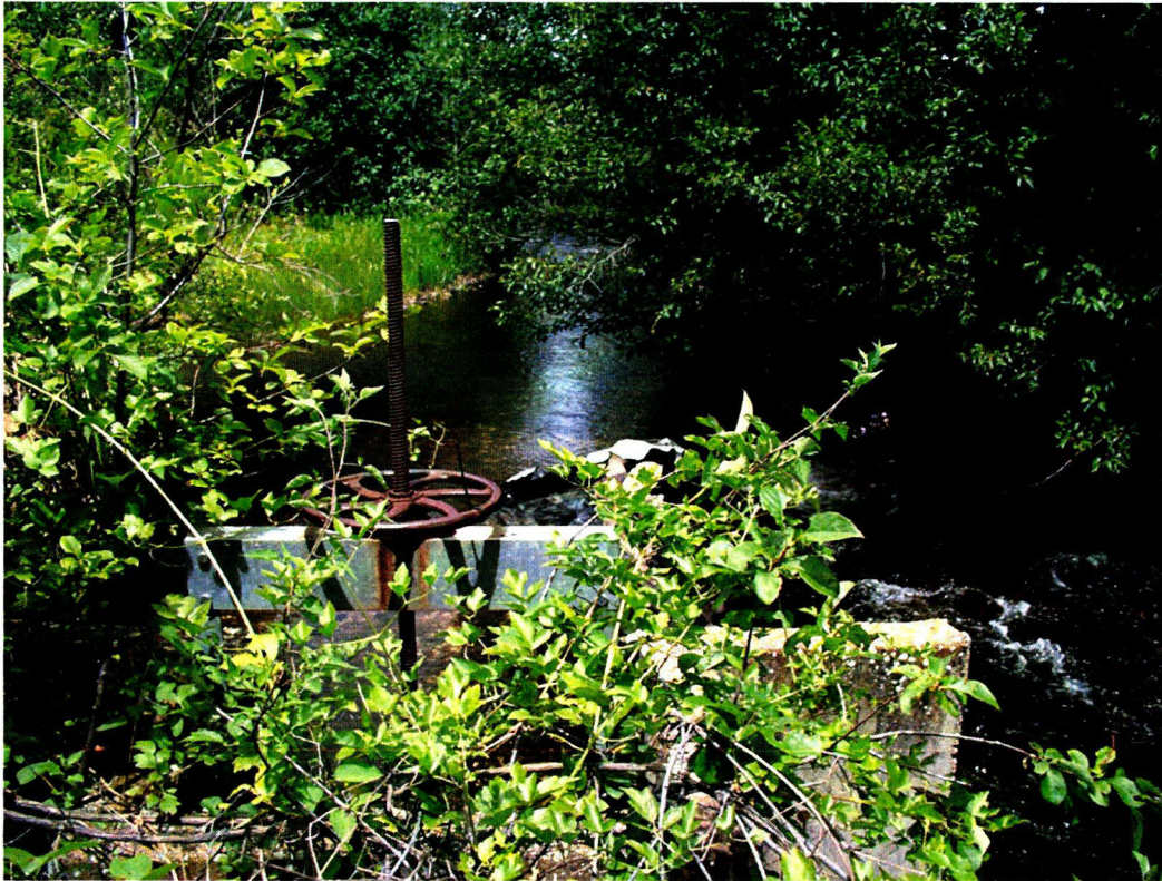
6/25/14 Pine Creek Diversion Inspection: Site #7 "Noah Upper Diversion" (Pine Creek) headgate.
