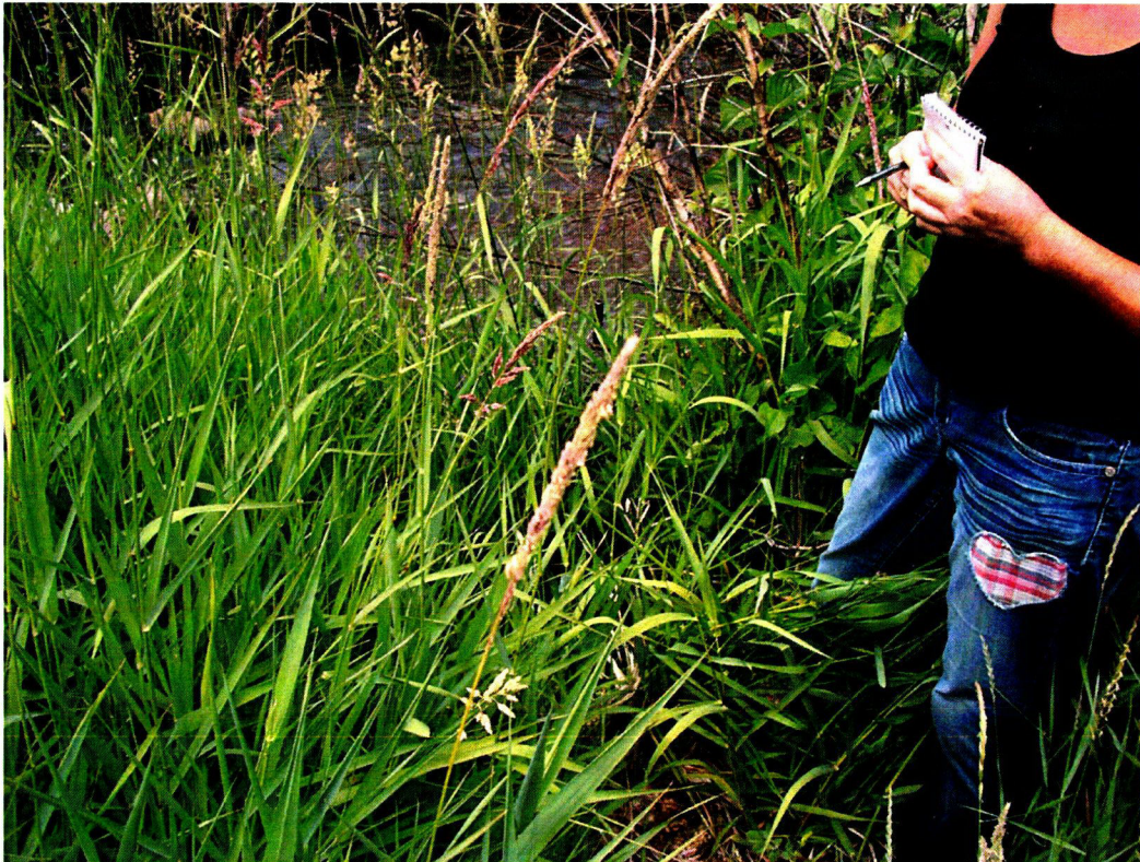
6/25/14 Pine Creek Diversion Inspection: Site #6 "Hansen & Weibe" (Pine Creek) headgate.
