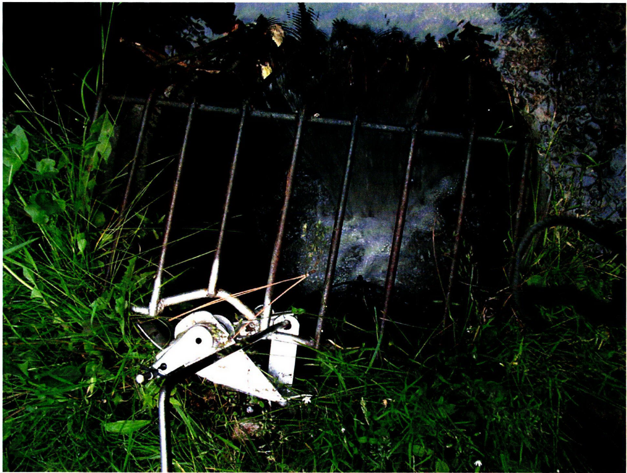
6/25/14 Pine Creek Diversion Inspection: Site #1 "Cuddy Meadows" (Little Pine Creek) headgate.
