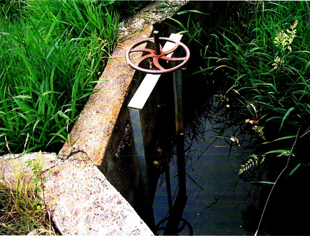
6/25/14 Pine Creek Diversion Inspection: Site #8 "Noah Lower Diversion" (Pine Creek) headgate.
