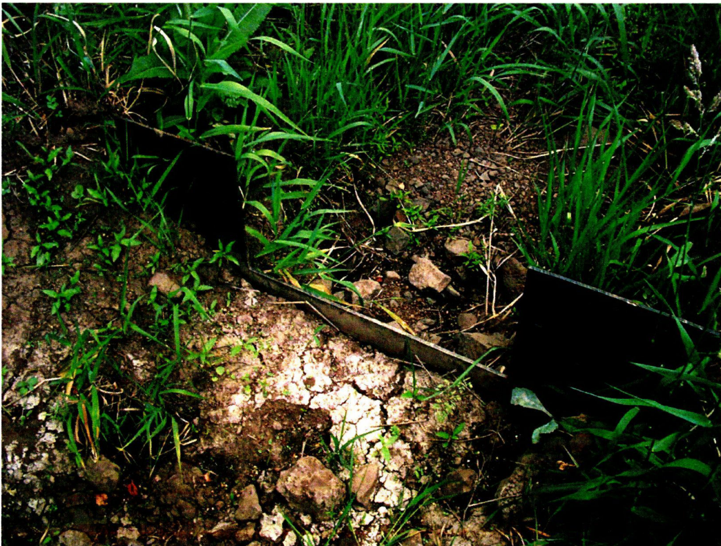
6/25/14 Pine Creek Diversion Inspection: Site #2 "Mink" (Pine Creek) measurement device.
