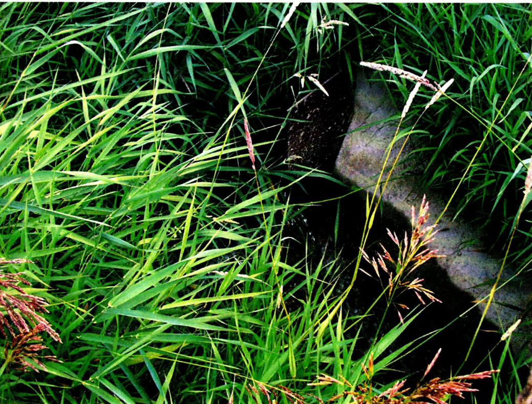
6/25/14 Pine Creek Diversion Inspection: Site #8 "Noah Lower Diversion" (Pine Creek) measuring device.
