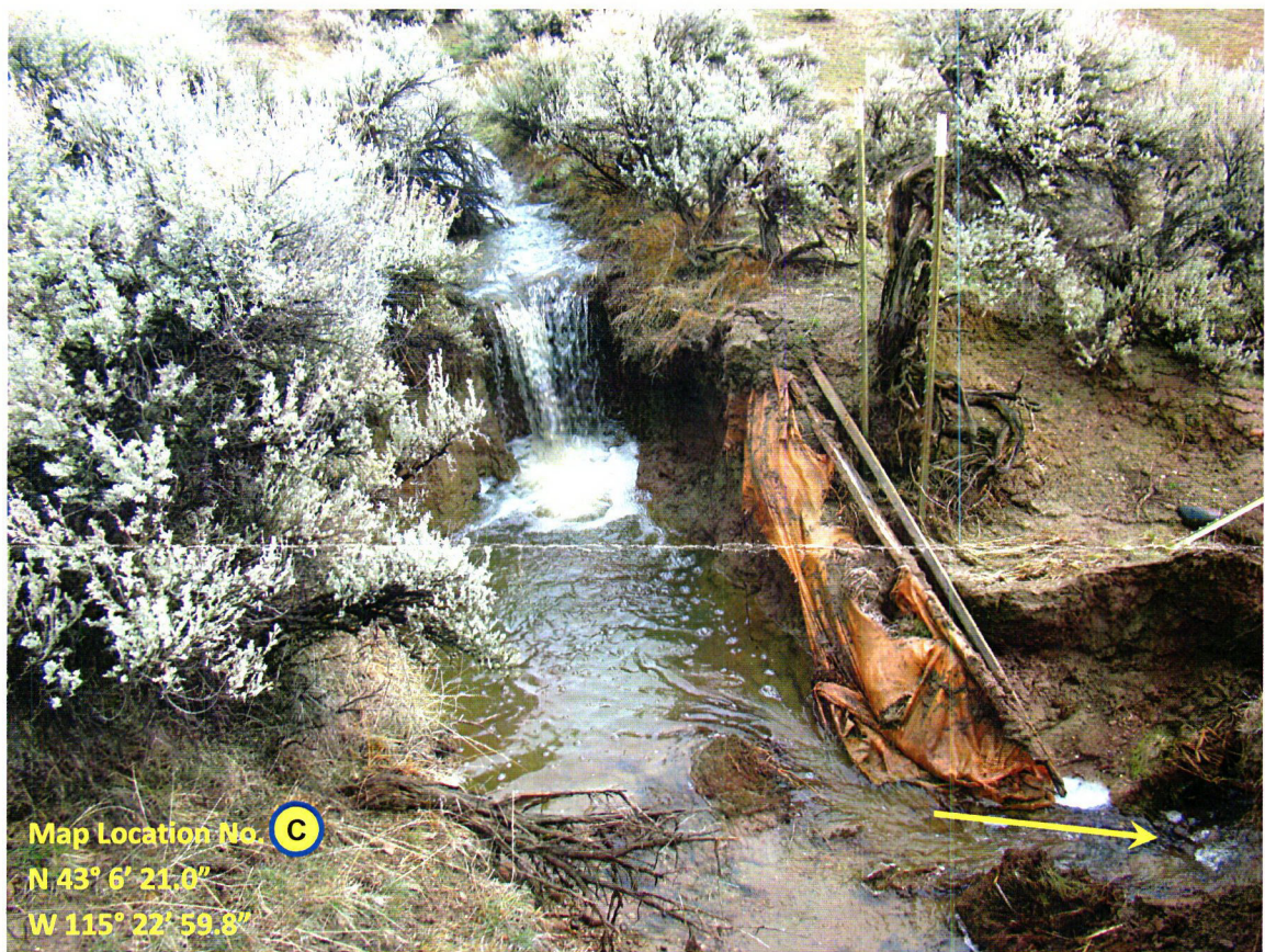
2-4-2015 photograph of the CDN “Four Mile Ditch” where it is breached (on right of photo) thus spilling ~ 3 cfs of surface water diverted from a Cold Springs Creek tributary into the Ryegrass Creek drainage (see Figure 1 for location No. C).
