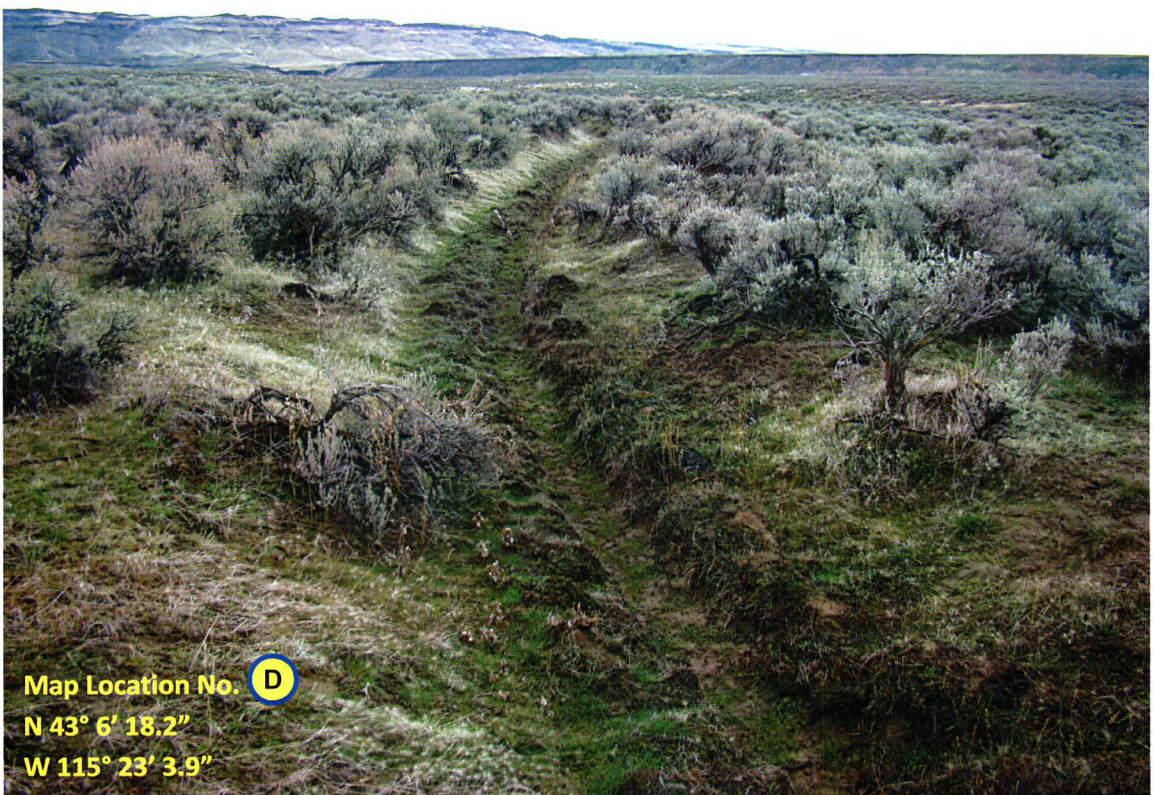
2-9-2015 photograph looking east along the dry Four Mile Ditch downstream of the “blow-out” shown on photo location No. C on the attached Figure 1. This portion of the ditch would have Cold Springs Creek water in it if the ditch was not breached as shown (See Figure 1 for location No. D).
