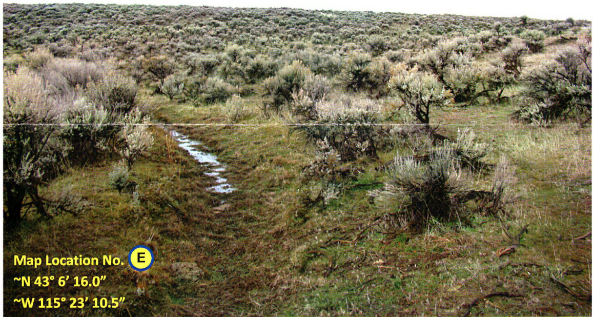
2-4-2015 photograph of slight standing water in the Four Mile Ditch from recent rains (see Figure 1 for location No. E). The ditch does not contain the flows from the Cold Springs Creek tributary at this point because of the blow out upstream.
