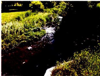
Off of 1050 East "Land Creek" 12 foot weir Note: The closure on both sides of creek approximately 14 feet down from weir.
