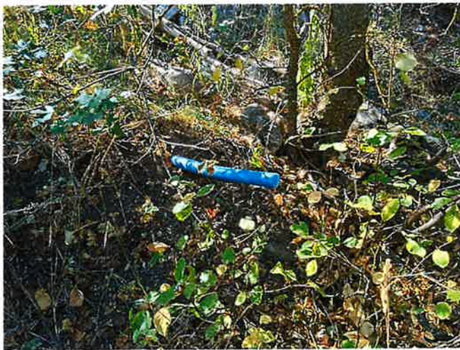
Drainage pipe (For clearing and cleaning system.)
