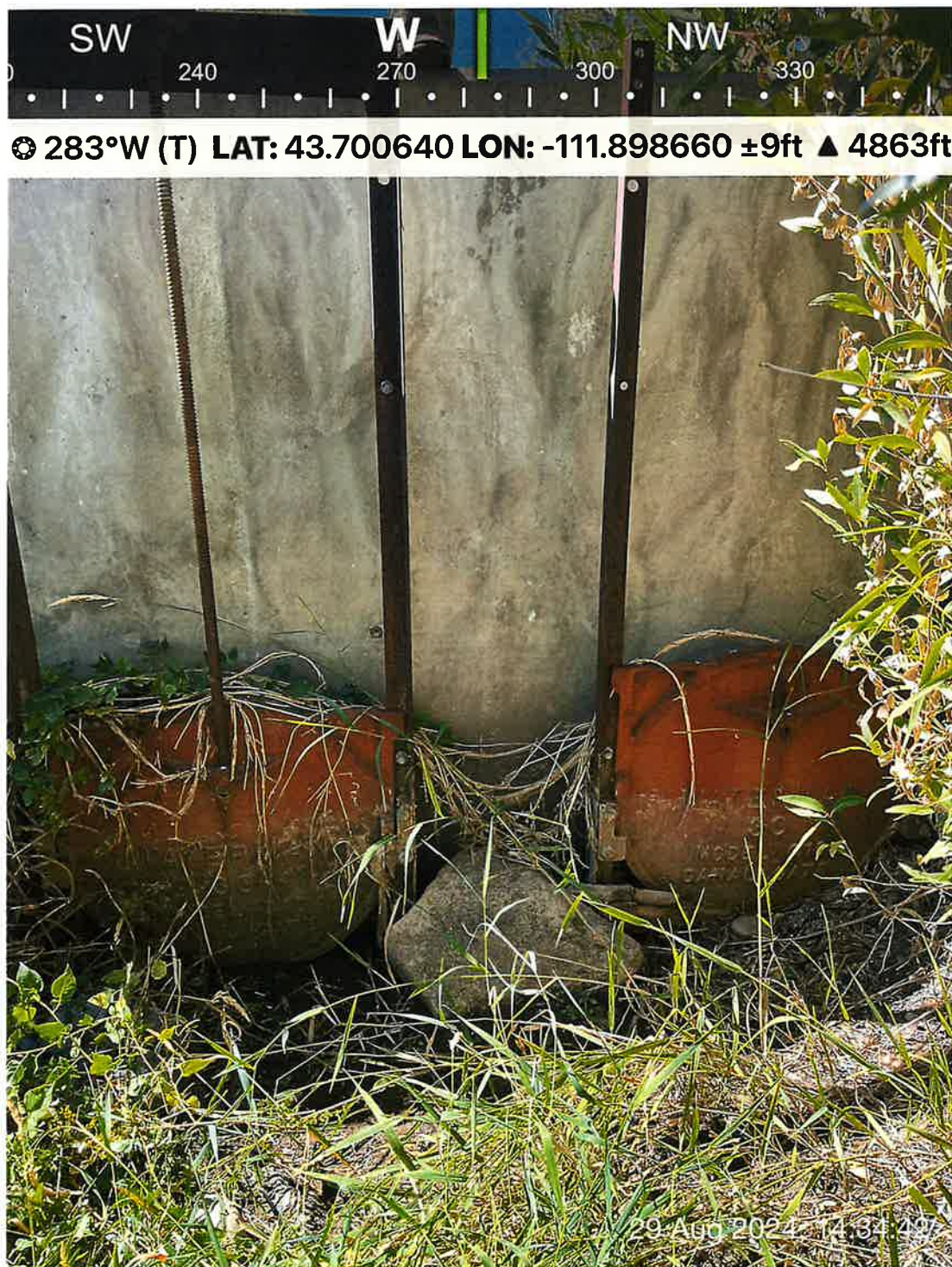
Headgate to the culverts going under the bridge.
