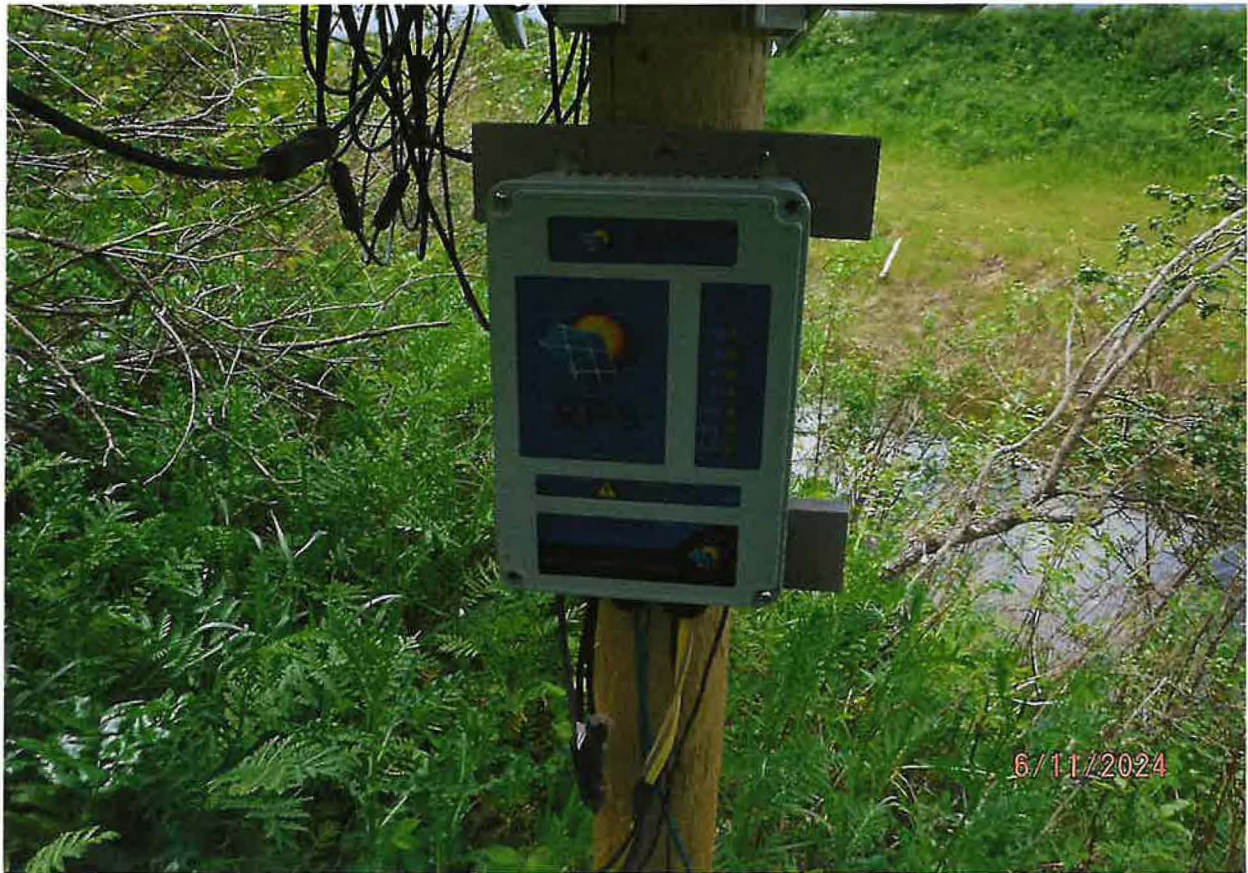
RURAL POWER SYSTEM SOLAR PUMP CONTROLLER
