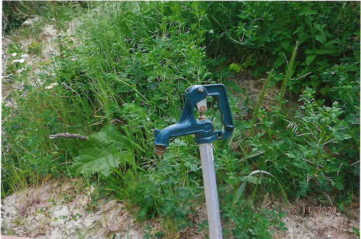
IRRIGATION & STOCKWATER POU – FROSTREE HYDRANT TO HOSE
