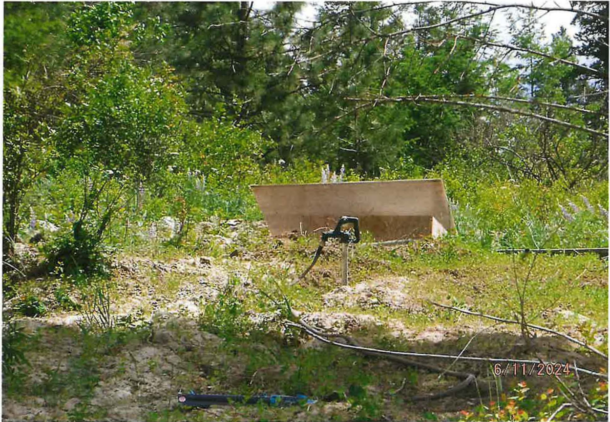
1,500-GAL VAULTED STORAGE RESERVOIR USES GRAVITY FLOW TO IRRIGATE BY HYDRANT(S) AND HOSES
