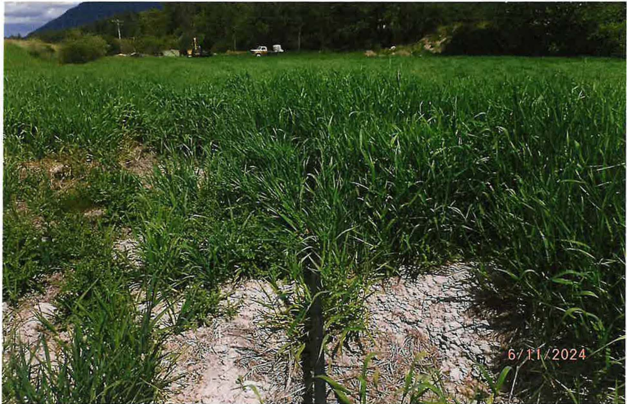
PIPELINE ROUTES ACROSS LOWLAND FIELD TO HILL SLOPE BUT DOESN'T EXTEND ALL THE WAY TO THE IRRIGATION POU
