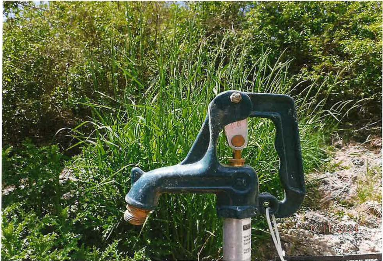
5-GAL BUCKET MEASUREMENTS TAKEN FROM FROST FREE HYDRANT
