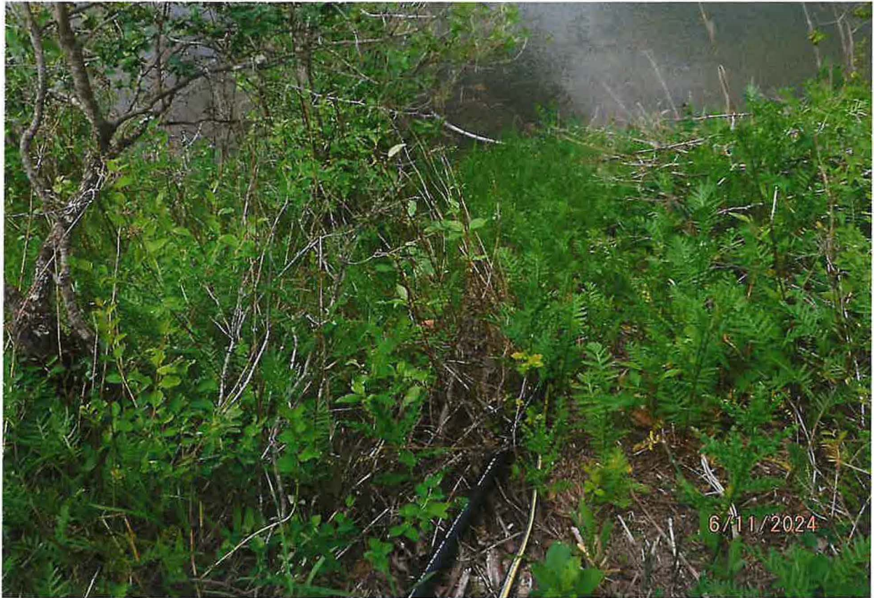
1-1/4 INCH POLYPIPE ROUTED UP STEEP EMBANKMENT FROM CREEK TO PUMP POWER SOURCE
