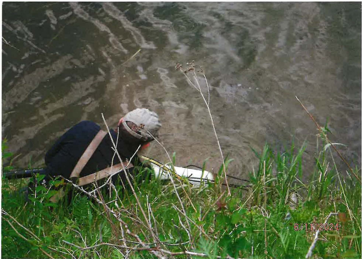
POD – SCREENED INTAKE PIPE DRAFTING WATER FROM MISSION CREEK
