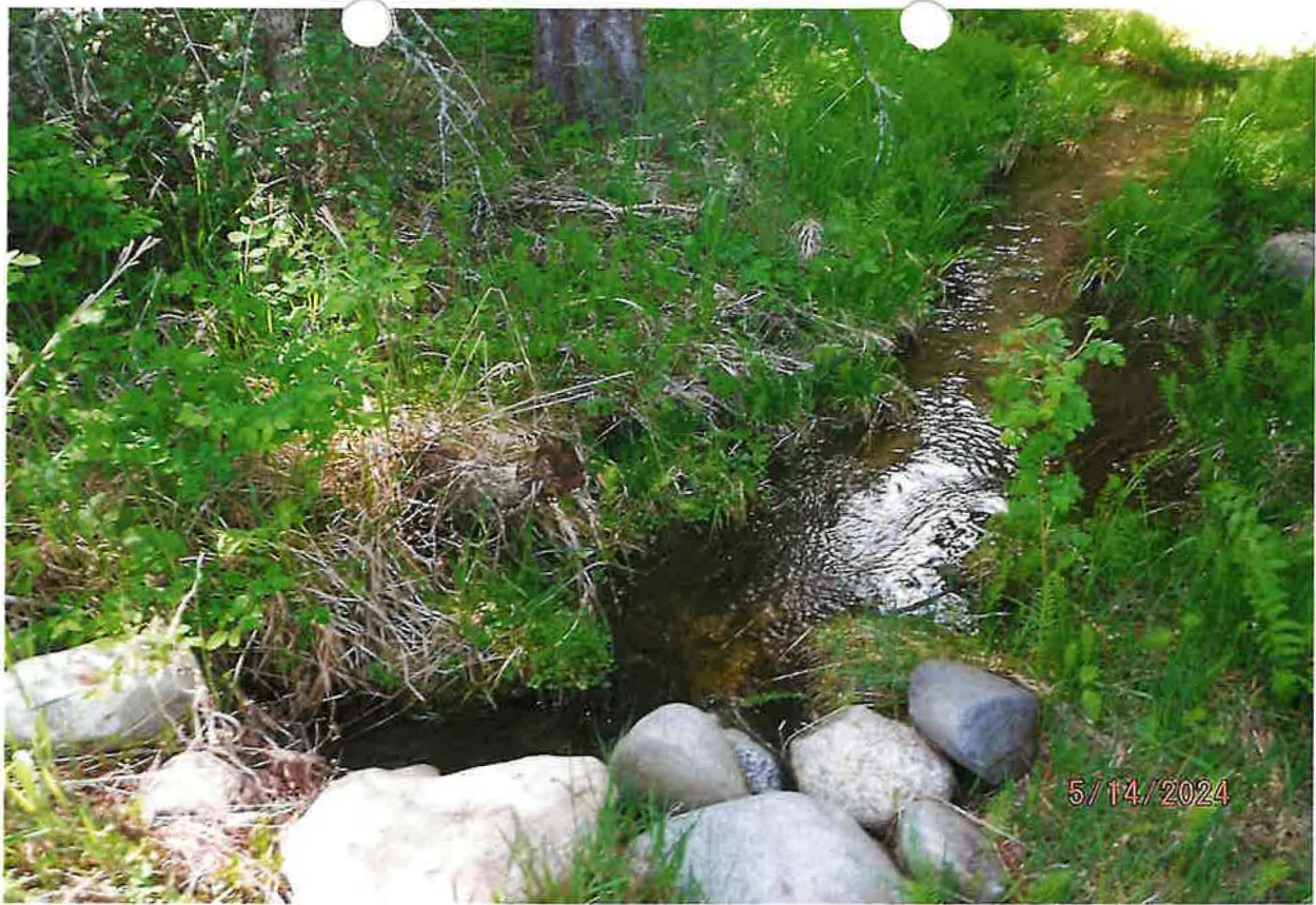
DIVERSION TO STORAGE – OPEN CONVEYANCE DITCH TRANSITIONS TO A SECOND RUN OF 8" CORRUGATED POLY PIPE WHICH FILLS THE STORAGE POND
