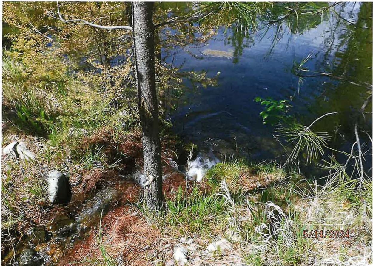
STORAGE POND OVERFLOW CHANNEL AS IT ROUTES TO THE 2 ND OF 5 TOTAL PONDS
