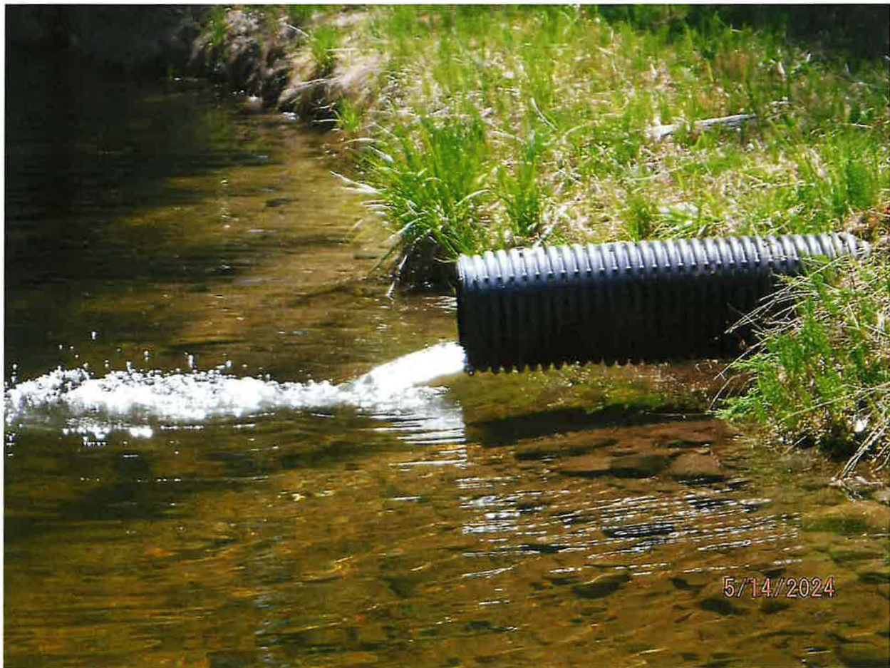
RECREATION (FLOW THROUGH WATER) POU – INFLOW TO POND FROM CONVEYANCE DITCH & PIPE CIRCULATES WATER WHICH OVERFLOWS BY EARTHEN CHANNEL TO LOWER GRADE POND(S)
