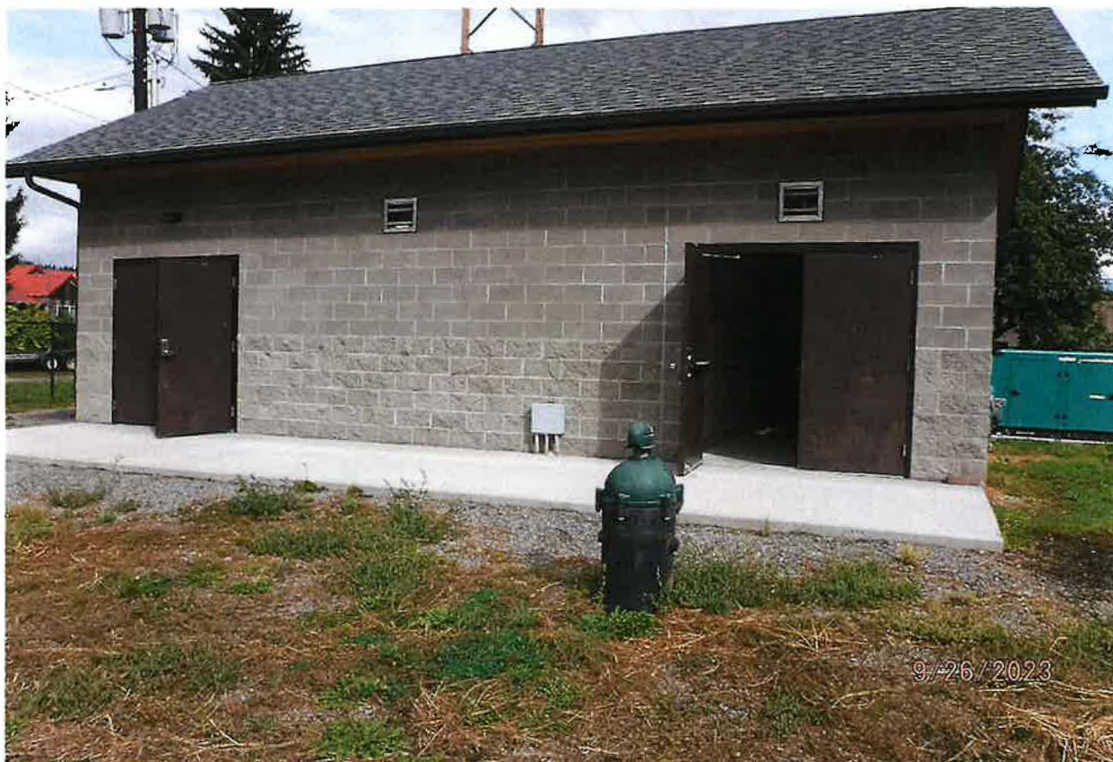
POD – GROUND WATER WELL D0079335
