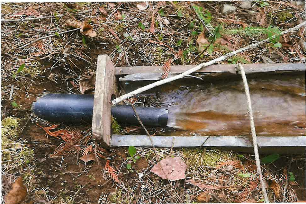
INFLOW FROM CONVEYANCE SYSTEM 1-INCH PIPE TO WOODEN RACEWAY TO UPPER STORAGE POND
