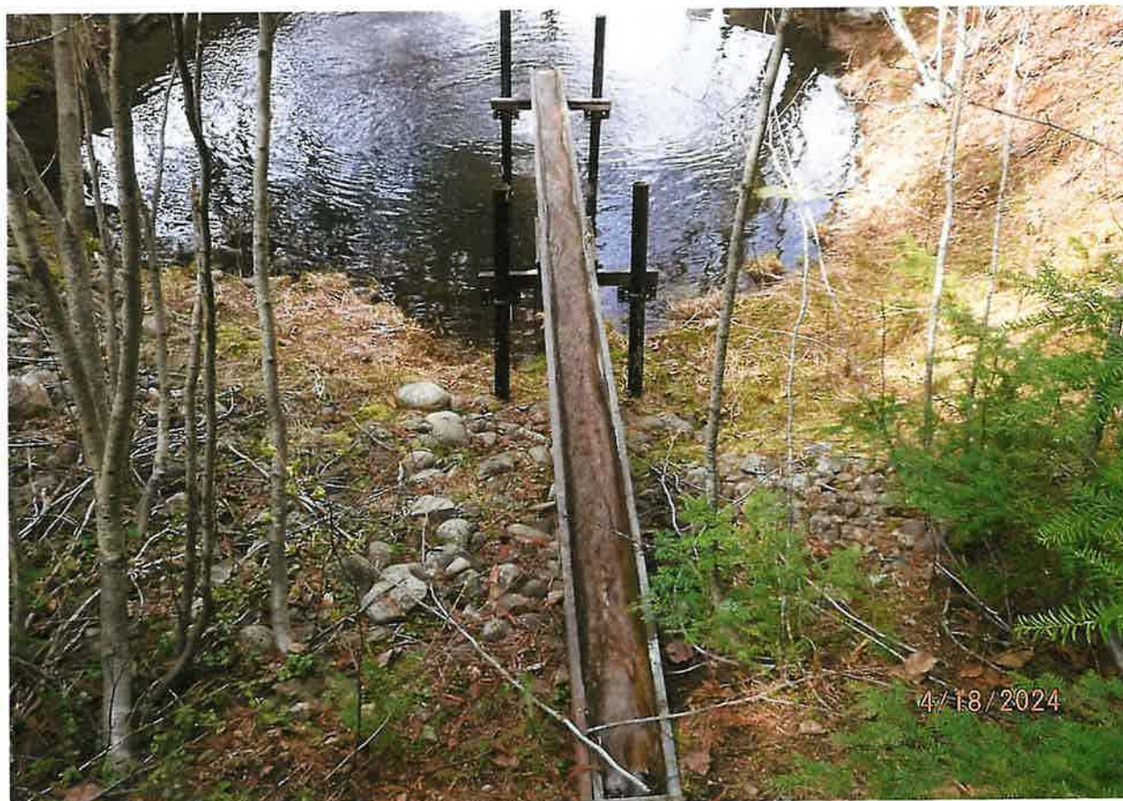
INFLOW FROM CONVEYANCE SYSTEM 1-INCH PIPE TO WOODEN RACEWAY TO UPPER STORAGE POND
