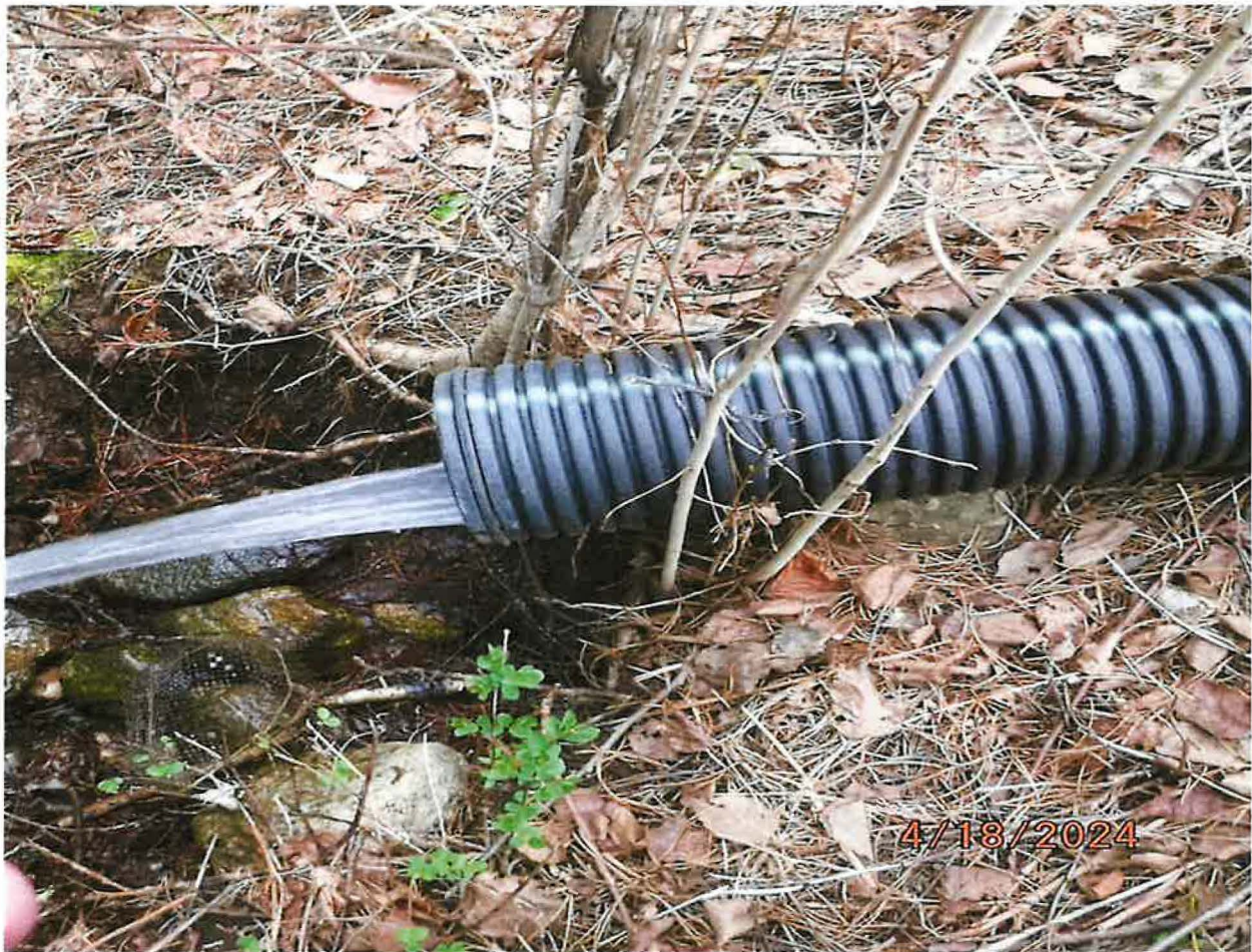
OVERFLOW WATER FROM LOWER POND DISCHARGES INTO A BURIED 120-FT RUN OF 6-INCH CORRUGATED PIPELINE THAT RETURNS UNNAMED STREAM WATER BACK TO THE SOURCE FROM TWO OFF-STREAM PONDS
