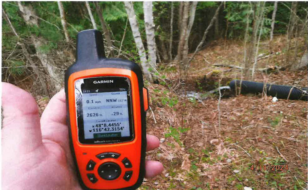
RECREATION POU – WATER FLOWS FROM POD TO TWO PONDS THEN RETURNS FLOW EXITING 6-INCH CORRUGATED DRAIN PIPE AND DOWN A SHORT EMBANKMENT BEFORE ADJOINING THE UNNAMED STREAM.
