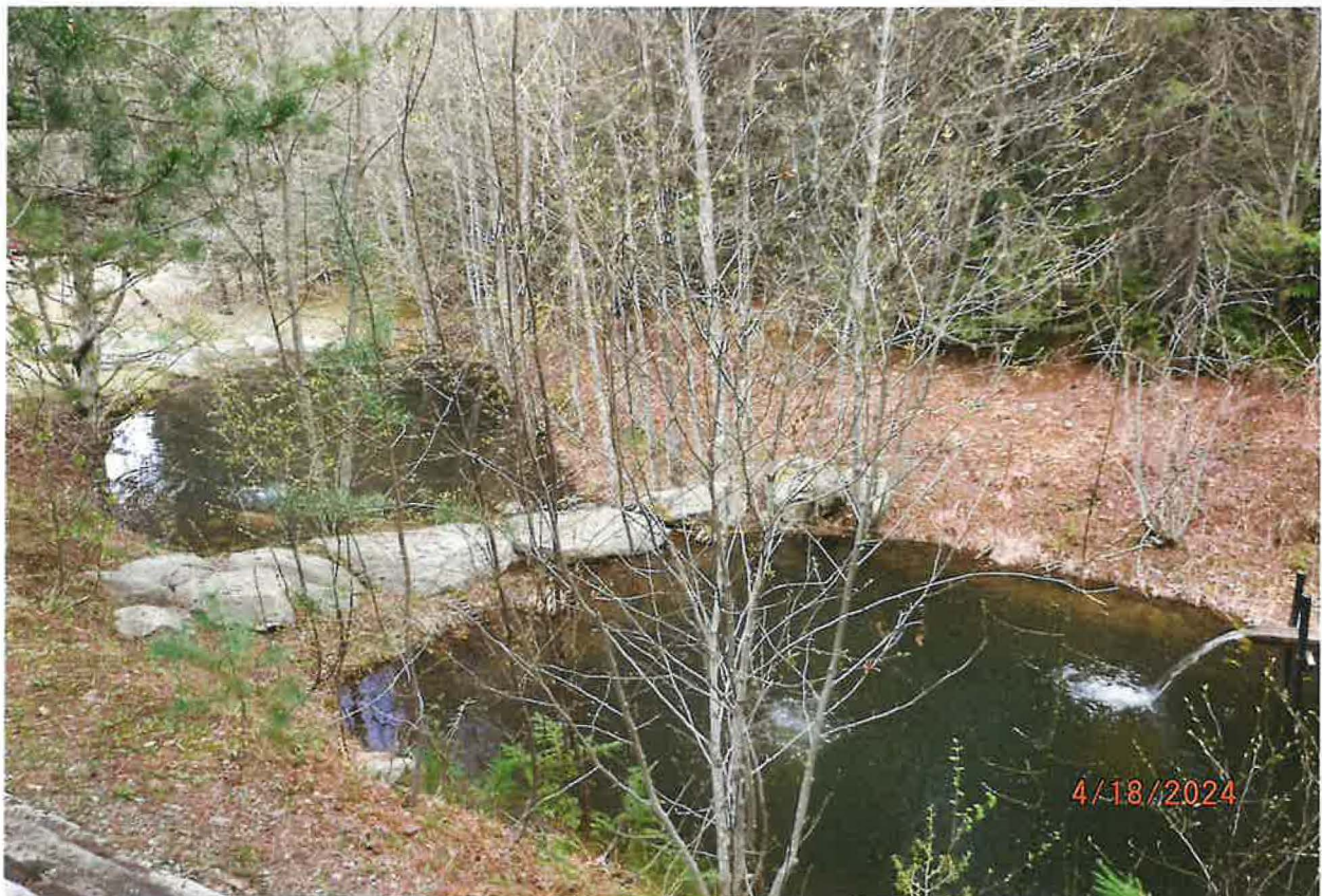
POU – 2EA STORAGE PONDS WITH SMALL EARTHEN DIKE AND FLOW THROUGH CHANNEL INTERCONNECTING THEM
