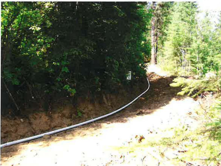
2" PVC water line instillation
