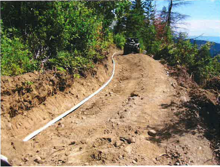
2" PVC water line instillation
