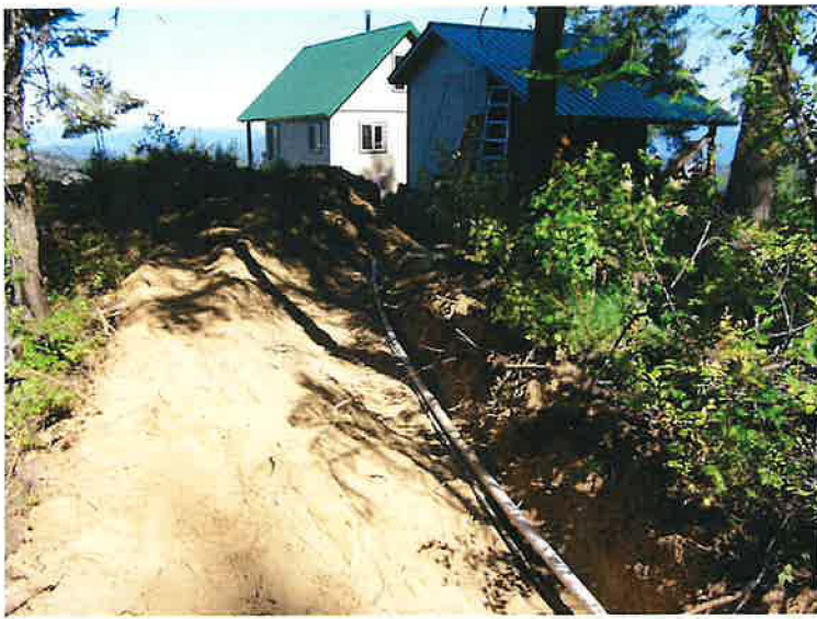
2" PVC water line instillation
