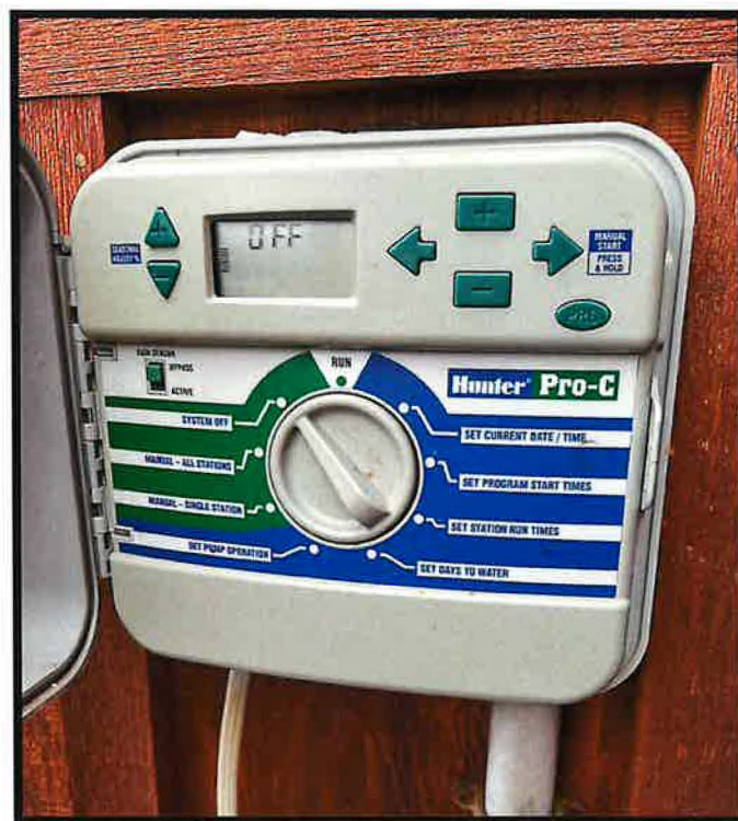
Photo 4- Irrigation Controller.
