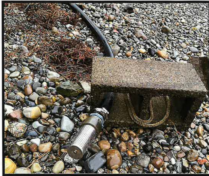
Photo 1- Intake screen and intake line.
