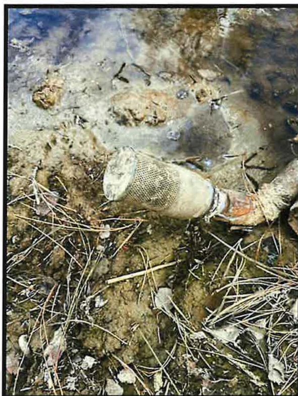
Photo 1 (left)- Hunter popup sprinkler head variations of which are used throughout the POU. Photo 2 (right)- Fish screen on the intake below the highwater mark of the lake.
