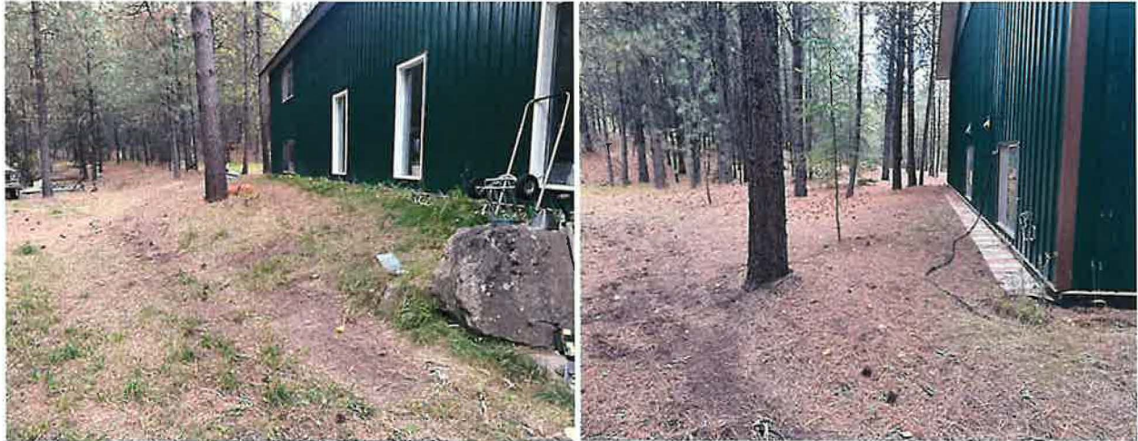
Photos 5 & 6- Area 3- Watered areas on the south and west sides of the shop, respectively. Note the hydrant located at the corner of the building in the photo on the right. Permit holder stated that is mostly to keep the area around the shop from drying out and becoming a fire hazard. This is not included in the domestic volume, as there is no evidence of irrigation.
