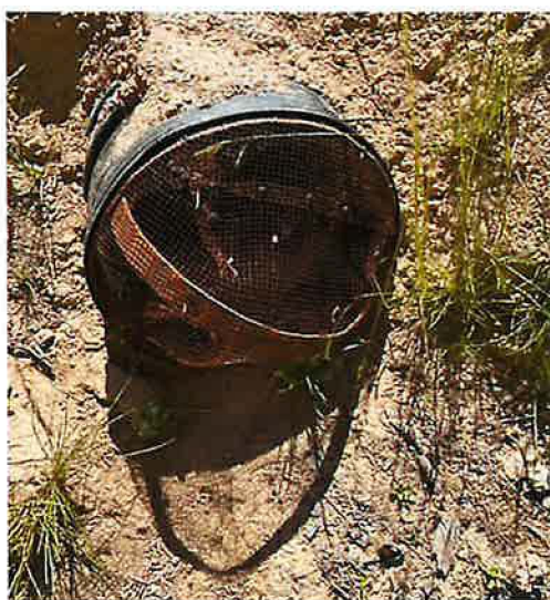
Figure 5: Northern pond screened outflow
