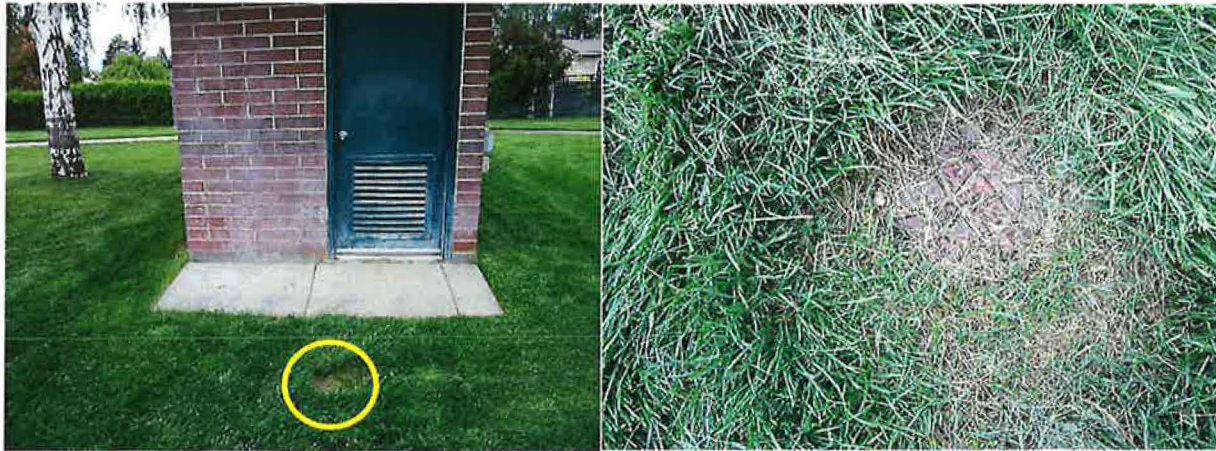
Figure 1b- Valve for diversion to the "Splash Pad".
