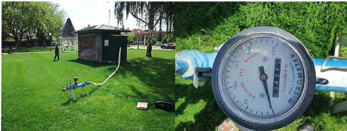
Figures 1.1 & 1.1a- Photo (facing east) of the pump house and measurement equipment as set up for measurements.
