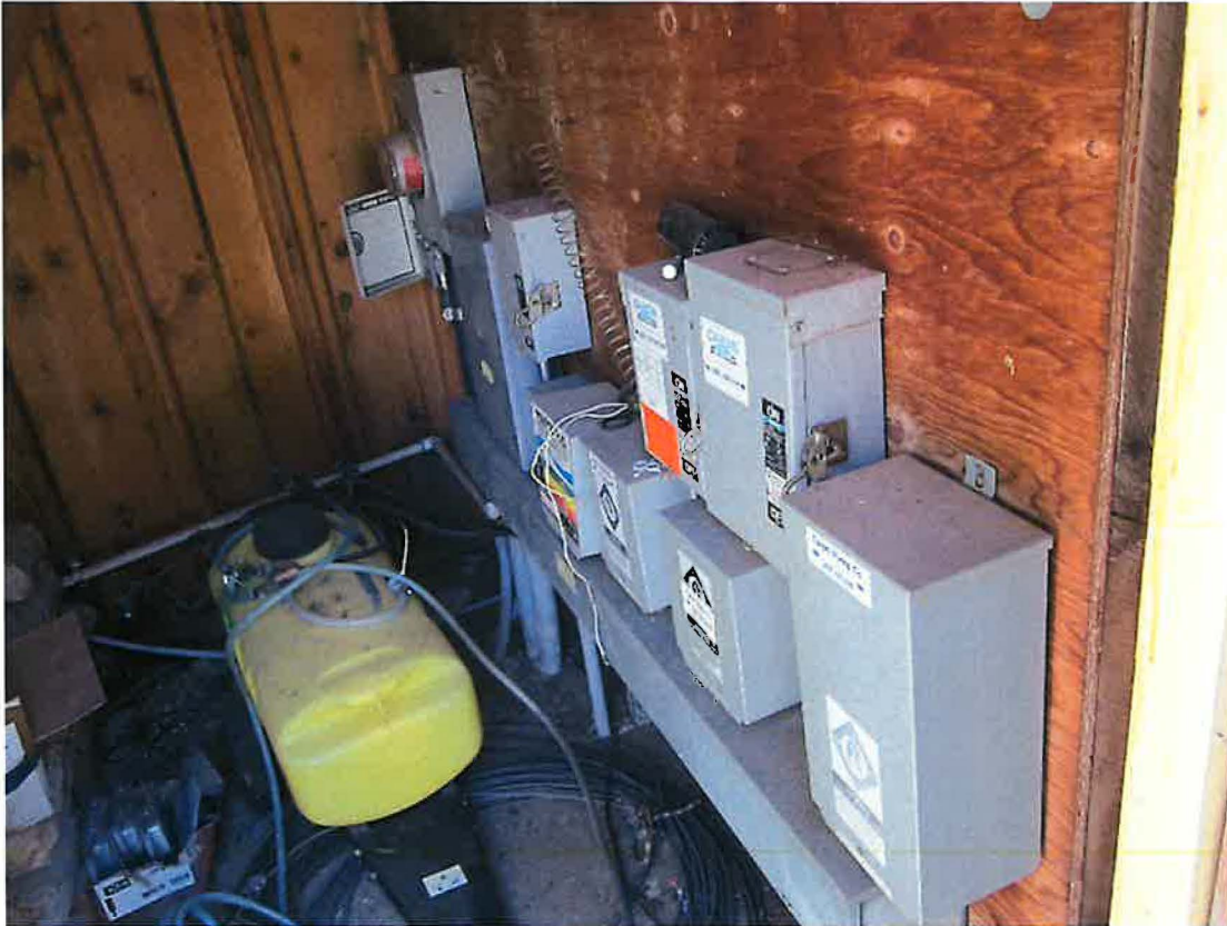
Photo 5- Power bank and pressure controls located inside of the pump house.
