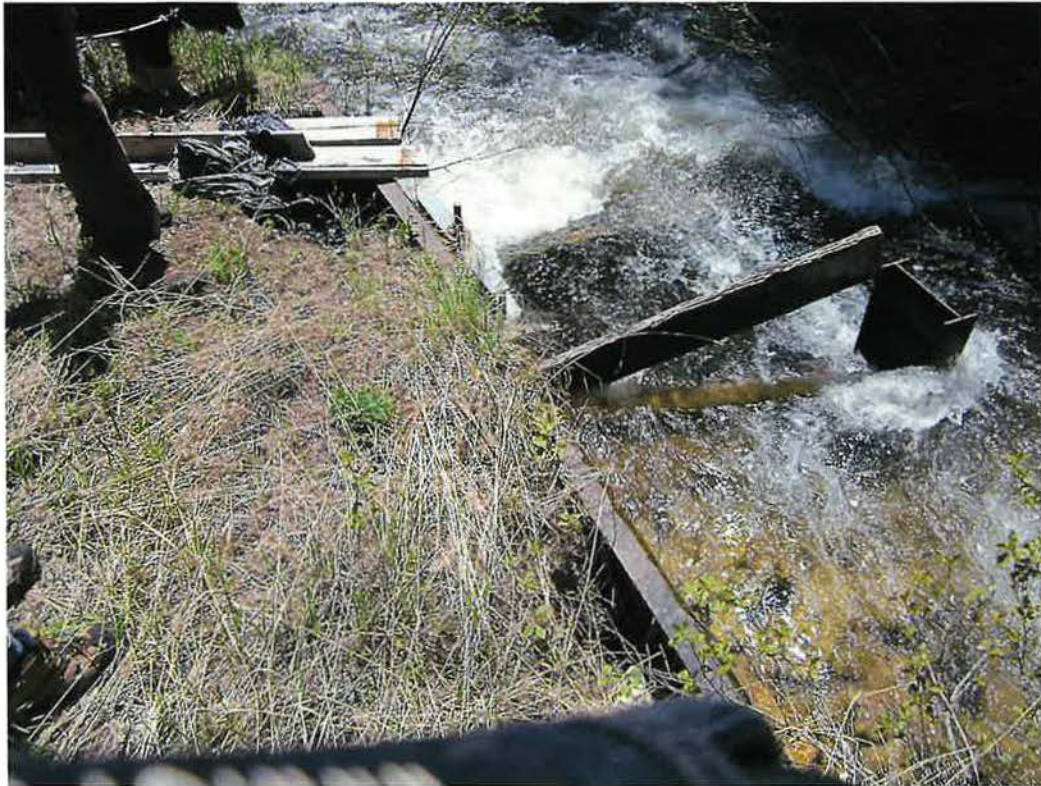
Photo 13- Head gate at Alder Creek, diverting water North into the irrigation ditch.
