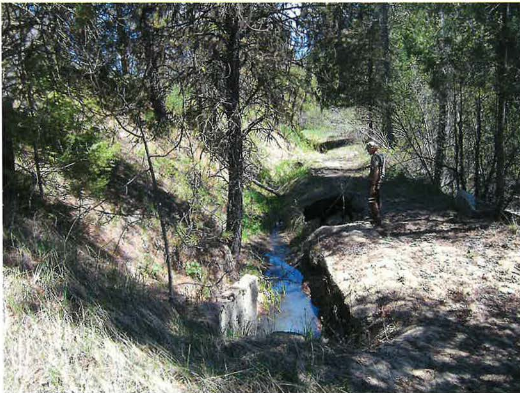
Photo 14- Irrigation ditch from headgate at Alder creek to the west side of the western pond.
