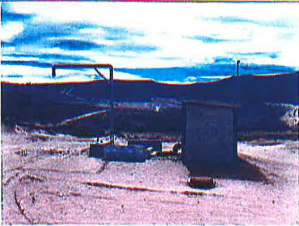
Photo 5: Manhole for 15,000 gallon concrete tank
